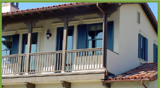
Extended balcony with heavy wood columns and corbel details; decorative window shutters and Mission profile roofs with extended overhangs.
