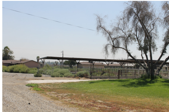
2. Existing dairy farm looking southeast.
