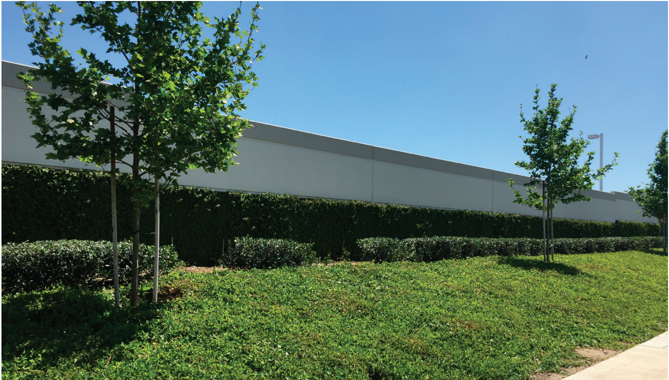
Photo 7.4 - Example of typical screen wall with landscaping
