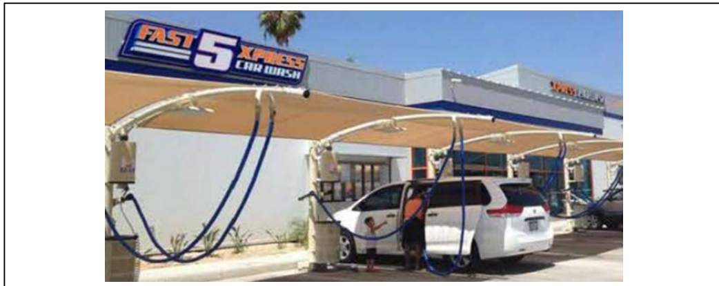
Figure 3: Vacuum Bay Canopy
