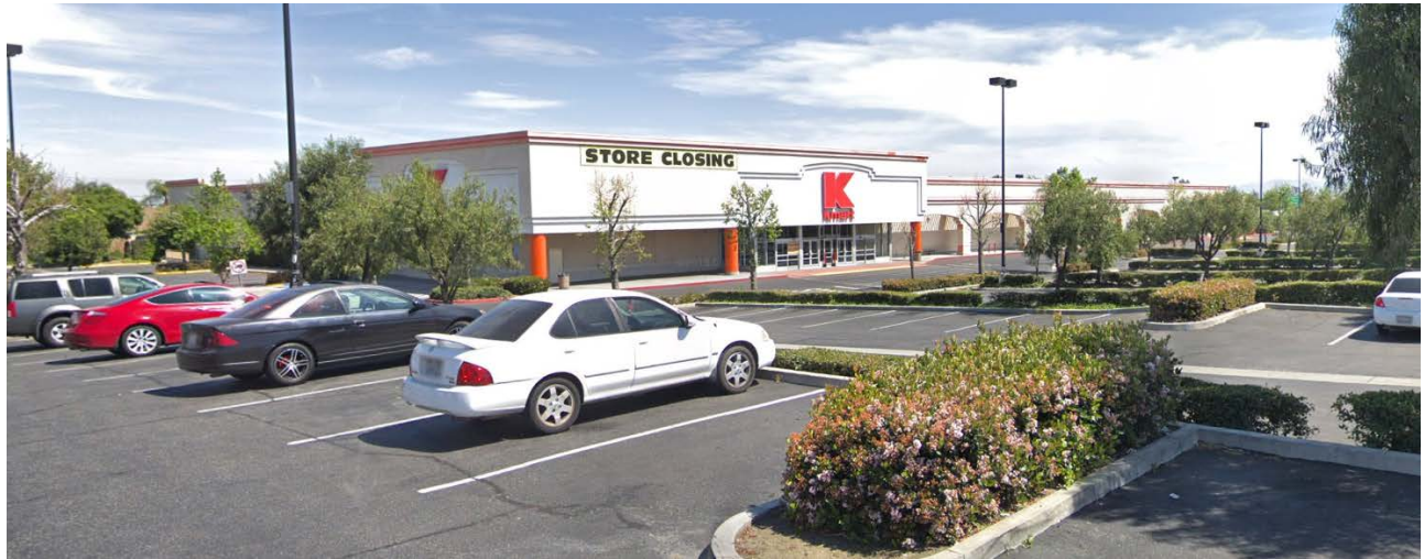
Northeast corner of existing commercial building (former K-Mart)
