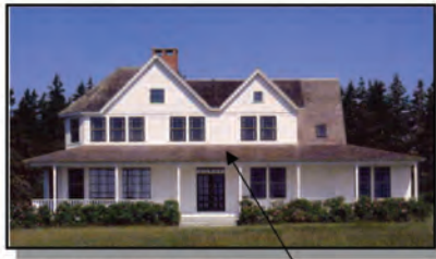
Porches along Front and Rear Elevations with a Shallow Roof Break
