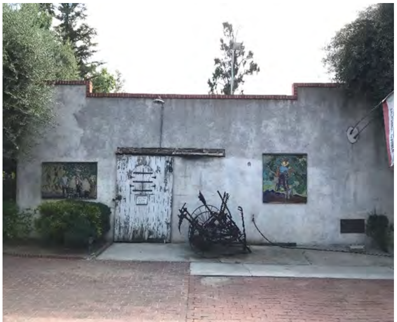
Image 4: West elevation of building, looking at the Museum entrance.
