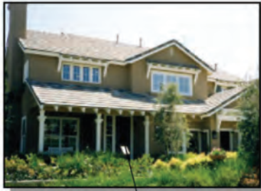
Stucco, Board and Batten and Horizontal Siding
