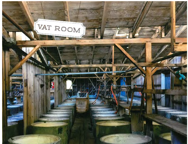
Image 7: Vat Room showing Vats (Resource No. 20).
