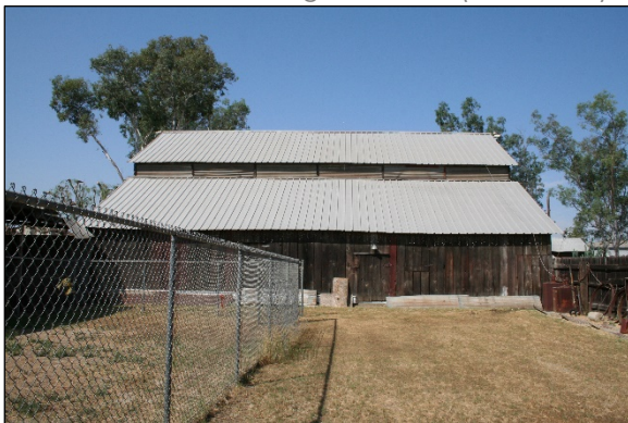
Figure 19: Barn, east (side) elevation, view facing west from corral (GPA, 2020)
