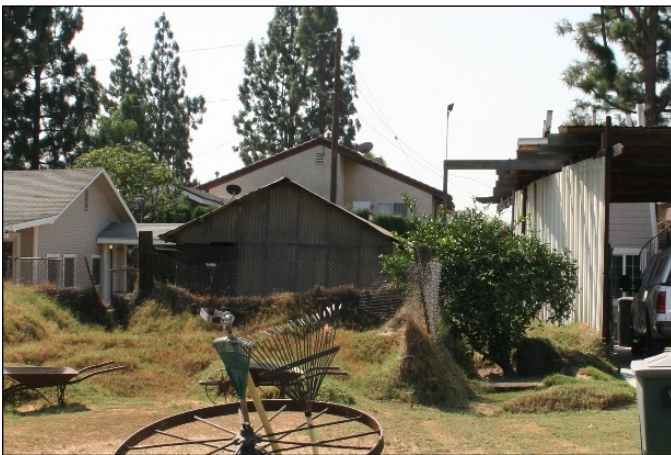
Figure 12: Garage, view facing south (GPA, 2020)
