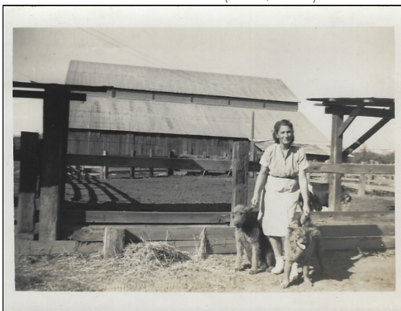
Figure 21: Barn, east (side) elevation, view facing west from corral c.1940s (Schmidt Family photograph)
