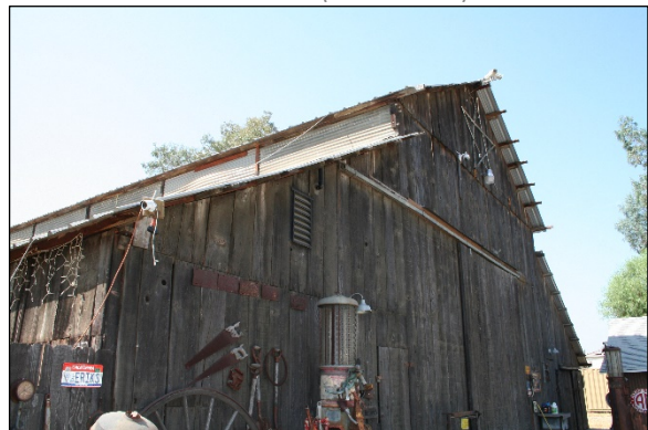
Figure 20: Barn, north (primary) elevation, view facing southwest (GPA, 2020)
