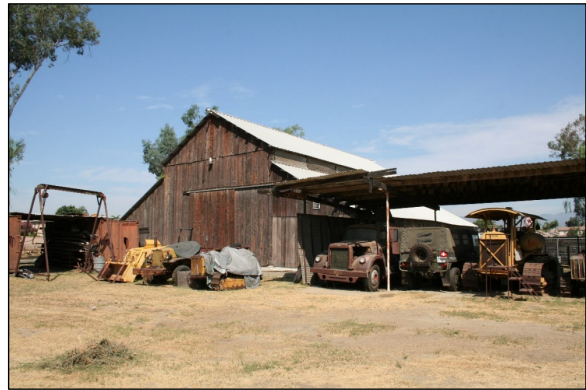
Figure 18: Barn, south (rear) elevation, view facing northwest (GPA, 2020)
