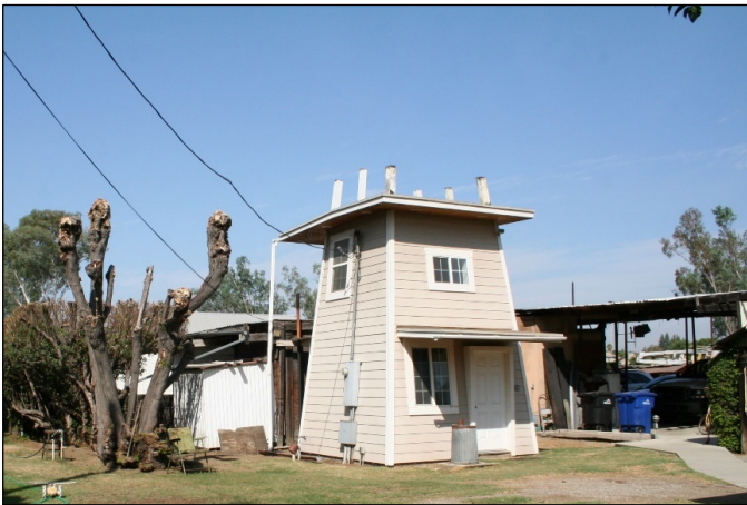
Figure 11: Pumphouse, view facing west (GPA, 2020)
