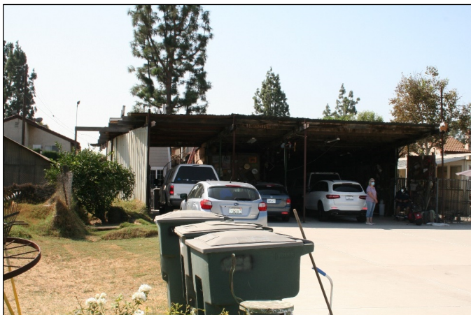
Figure 13: Carport, view facing southwest (GPA, 2020)
