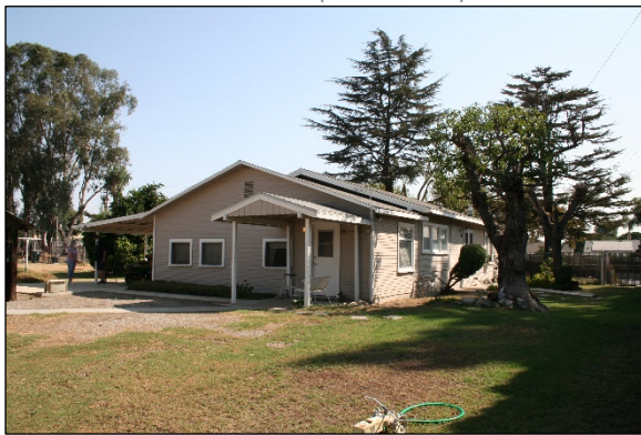
Figure 8: Residence, rear elevation, View facing northeast (GPA, 2020)
