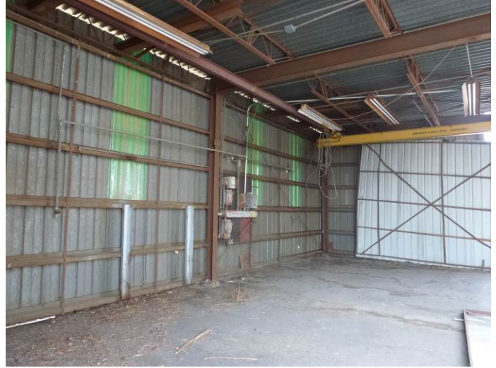
Image 14. Interior view of the Wash Building.
