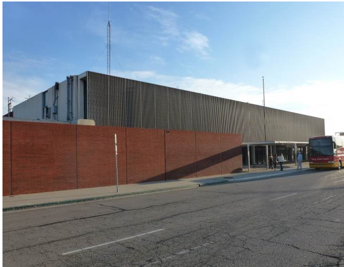
Image 3. View looking south at the northeast and northwest façades.
