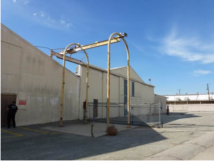
Image 5. View looking west at the northeast façade.
