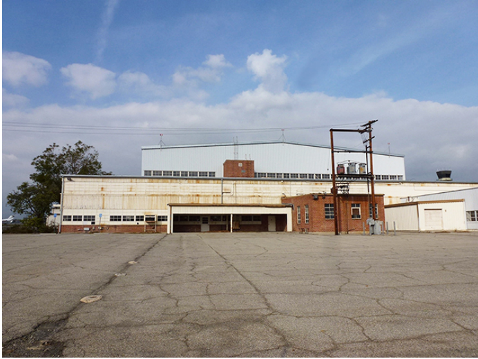
Image 5. View looking north at the south façade.
