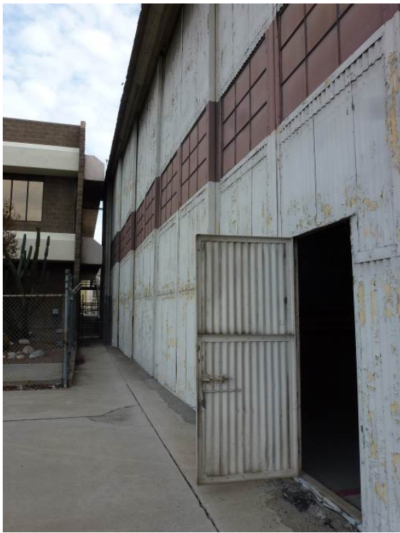
Image 3. Detail view looking at the northwest façade.
