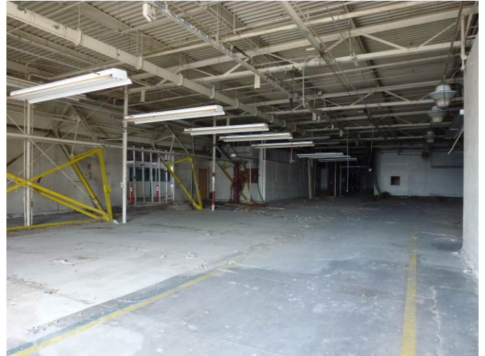
Image 4. View of the interior looking southwest.
