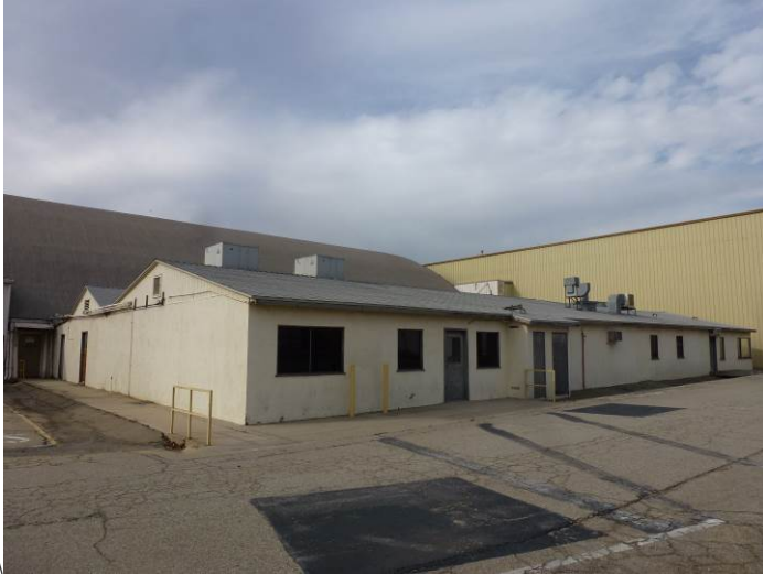
Image 9. View looking north at the southwest and southeast façades of the Commissary Building.
