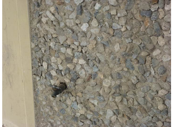
Image 2. Detail view of aggregate concrete panel.
