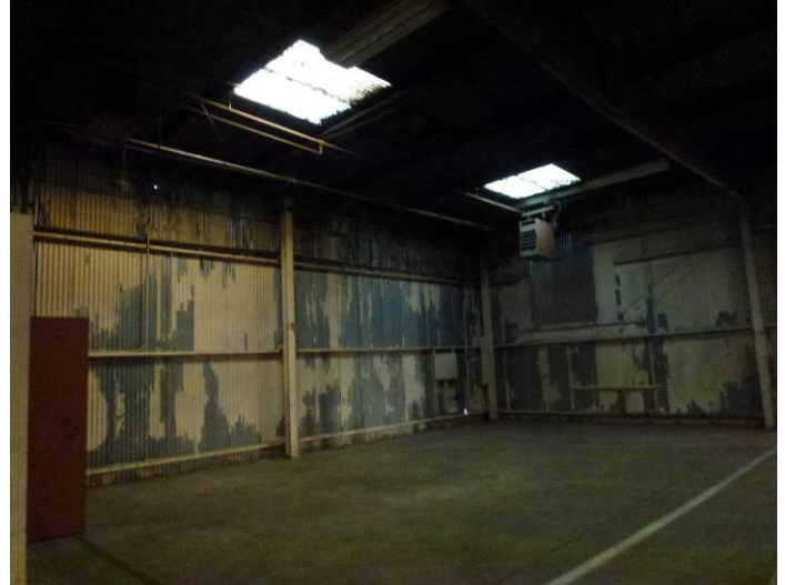
Image 6. Interior view of south wing.
