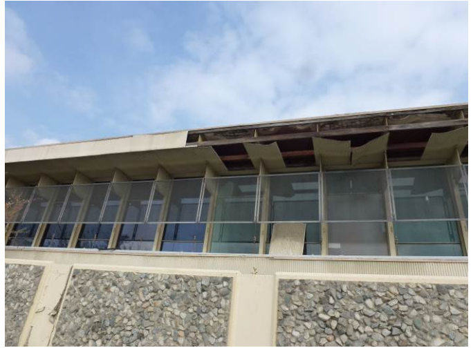
Image 6. Detail view of the south façade.
