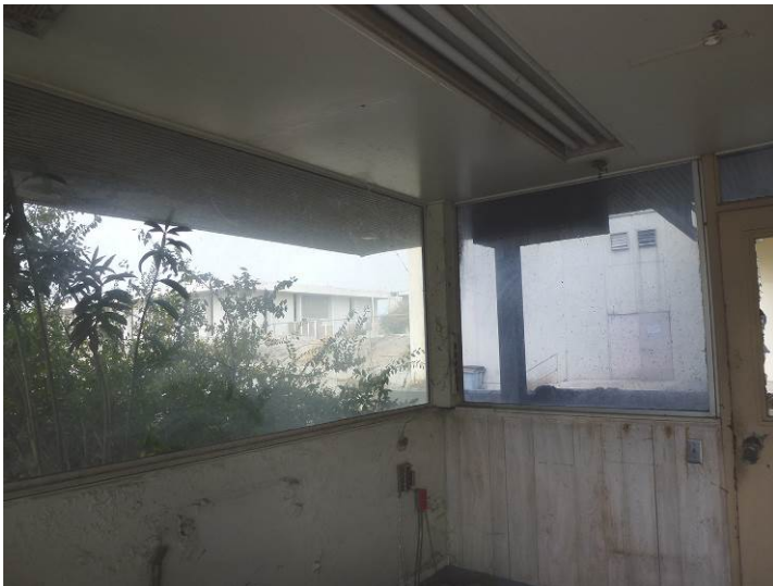
Image 3. From the interior looking northwest.
