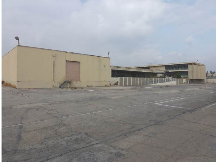
Image 1. View looking northwest at the west and east façades of buildings 12, 11, and 10.
