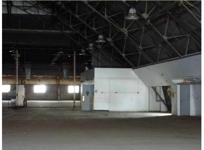
Image 6. Interior view looking southeast.
