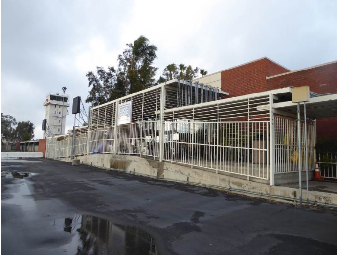
Image 5. View of Control Tower looking west from runway. As a later addition to the terminal, this portion of the building does not contribute to the historical significance of the building.
