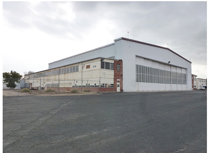
Image 4. View looking southwest at the east and north façades.
