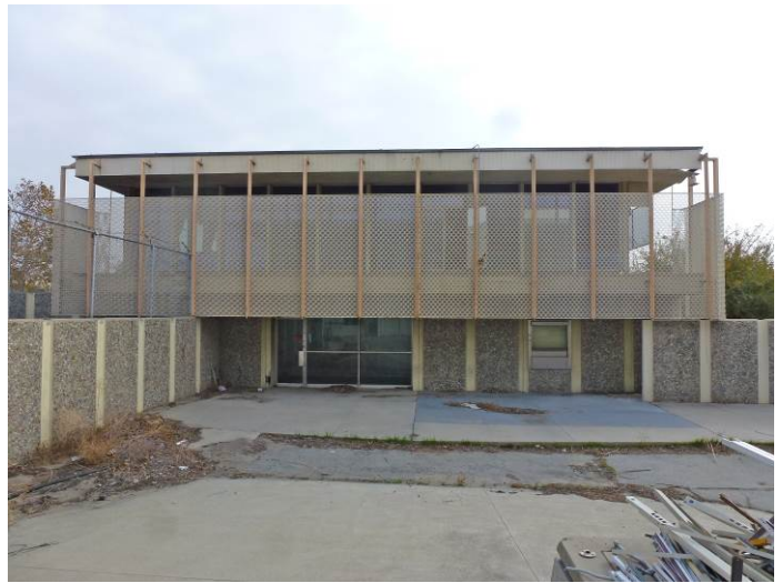
Image 2. View looking east at the west façade.
