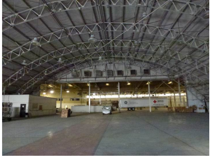
Image 2. Interior view looking northwest.
