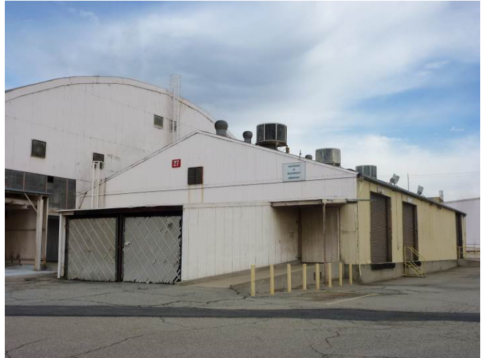
Image 6. View looking north at the southwest and southeast façades of Building 27.
