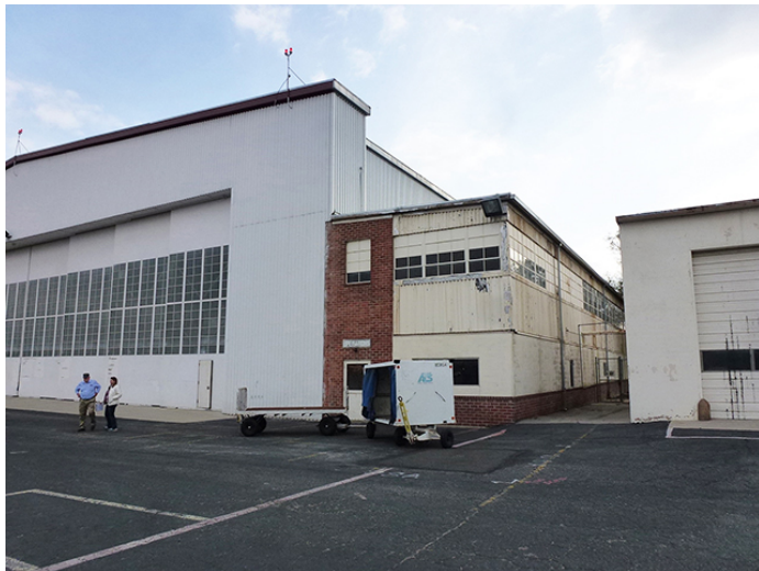
Image 3. Detail view looking southeast at the north and west façades.
