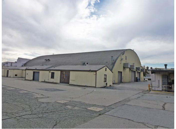
Image 2. View looking south at the northwest and northeast façades of Hangar 4 and Building M.
