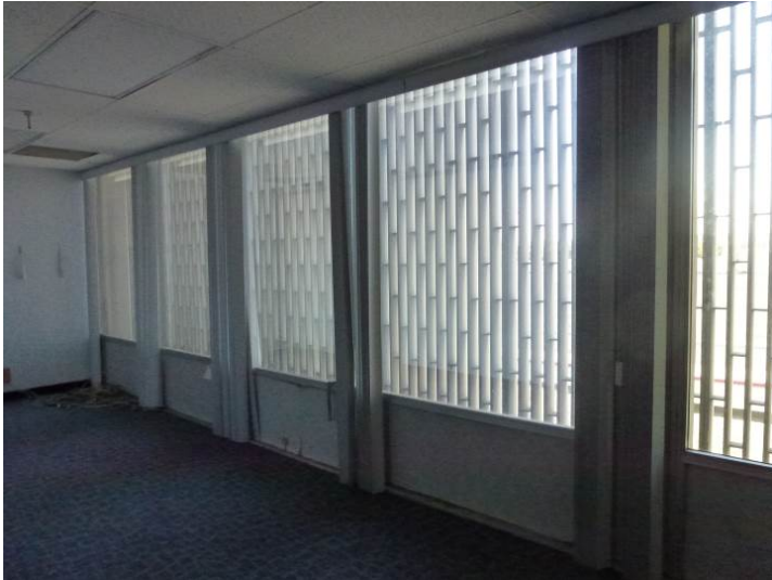
Image 9. Interior view of second-floor offices.
