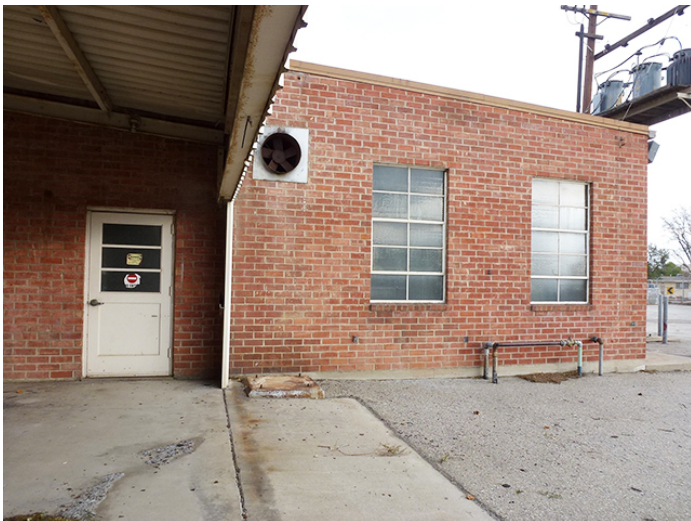
Image 7. Detail view looking east at the west façade of the Diesel Tanks room.
