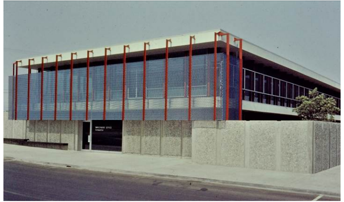
Image 10. View looking northeast at the west and south façades, ca. 1956. Source: Collection of Colin Russell.
