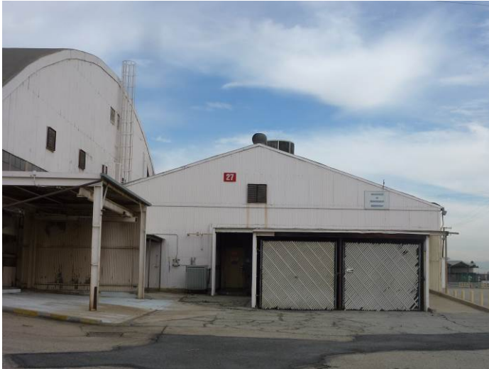
Image 5. View looking northeast at the southwest façade of Building 27.
