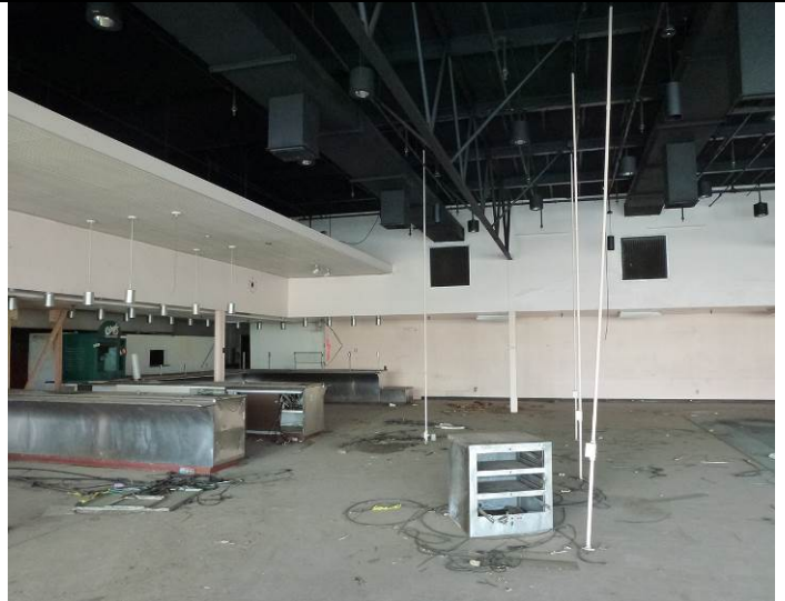
Image 4. Interior view looking southwest.
