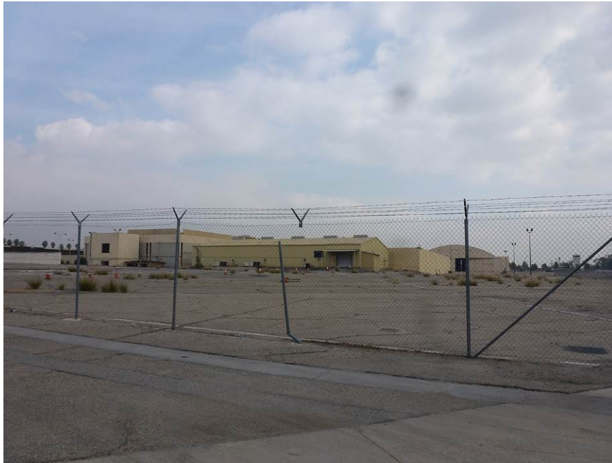
Image 5. View looking northwest at the LAS facilities.
