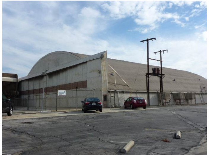
Image 2. View looking east at the northwest and southwest façades.
