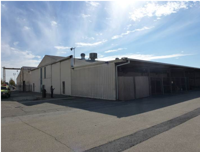
Image 3. View looking south at the northwest and northeast façades.
