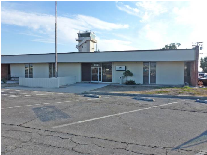
Image 6. View looking south at the north façade of the FAA building. This building is recommended as a contributor to the historic district.
