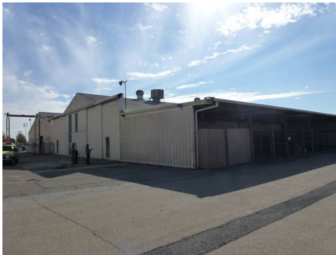
Image 3. View looking south at the northwest and northeast façades.
