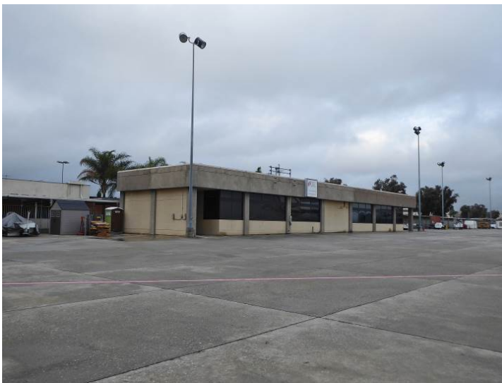
Image 19. View looking north from the runway area at the southwest and southeast façades of one of the holdroom (gate) buildings. As later additions to the terminal, these portions of the terminal do not contribute to the historical significance.
