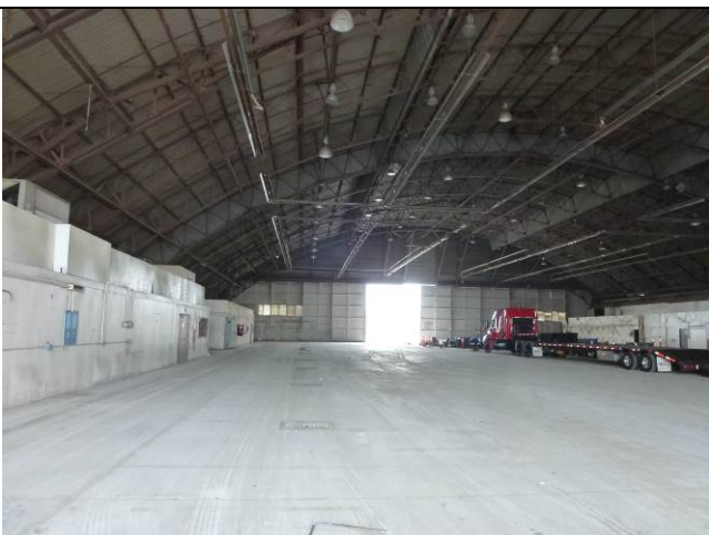
Image 5. View of the interior looking west.
