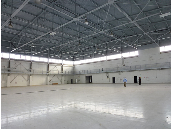
Image 13. Interior view of the hangar looking southeast.
