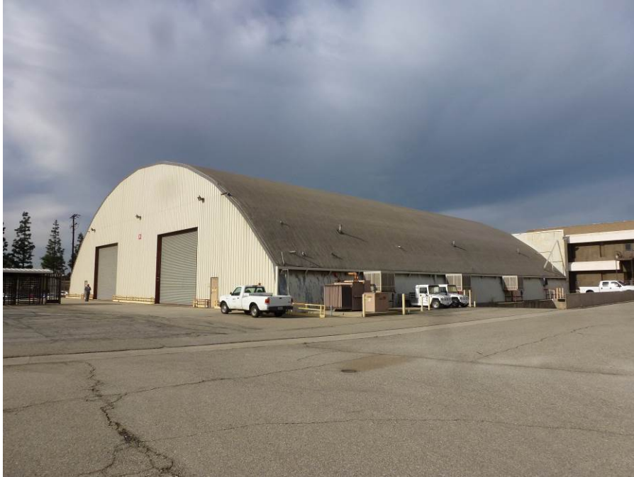
Image 1. View looking west at the southeast and northeast facades of Hangar 7 with the administration building to the right. ASM, December 1, 2016.
