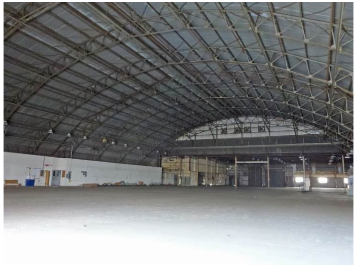
Image 4. Interior view of Hangar 4 looking southeast.
