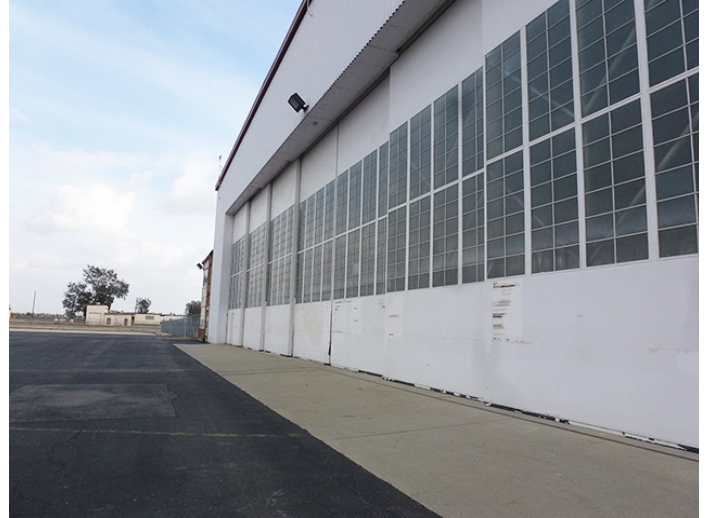
Image 2. View looking east at the west façade.
