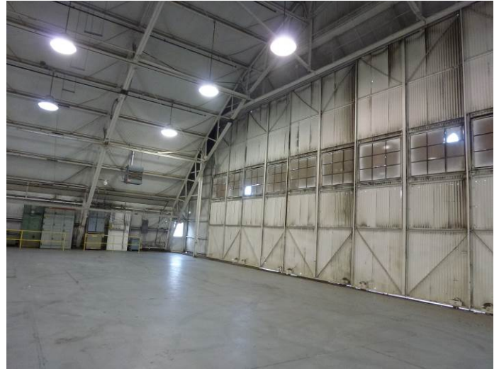
Image 6. Detail view of the interior looking west.
