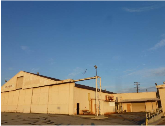
Image 1. View looking northeast at the west and south façades.
