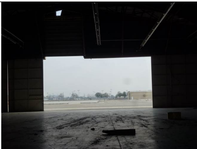
Image 5. View from the interior looking east.
