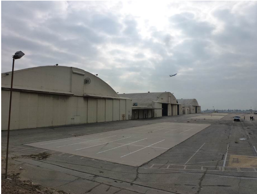
Image 3. View looking southeast at the west and north façades of hangars 6, 4, and 2.
