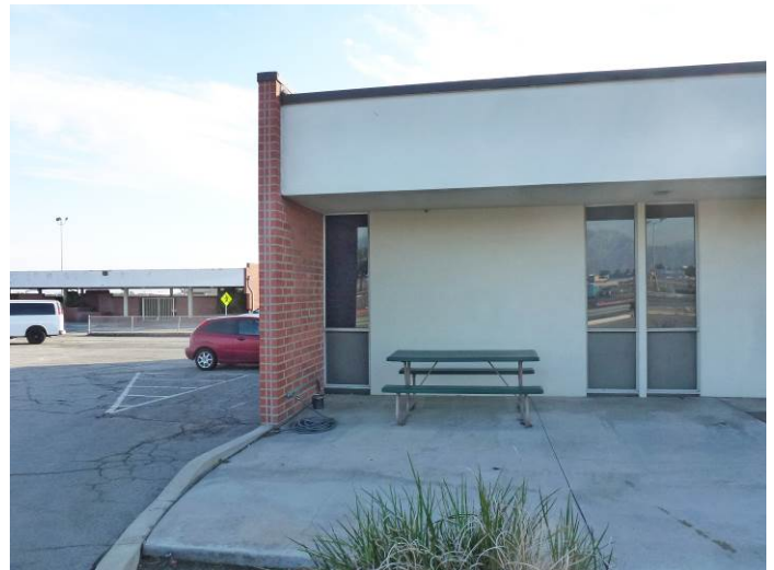
Image 4. Detail view looking at the north façade.
