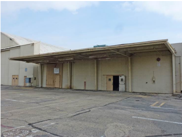
Image 1. View looking northeast at the west façade.
