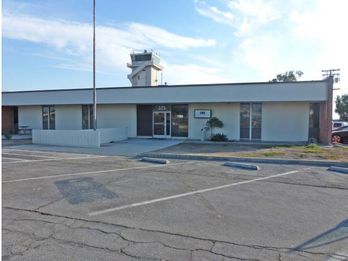
Image 1. View looking south at the north façade.
