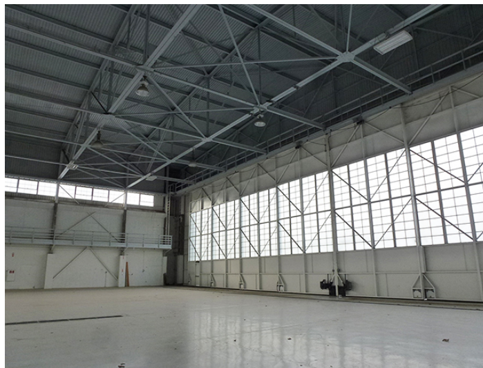
Image 11. Interior view of the hangar looking northwest.
