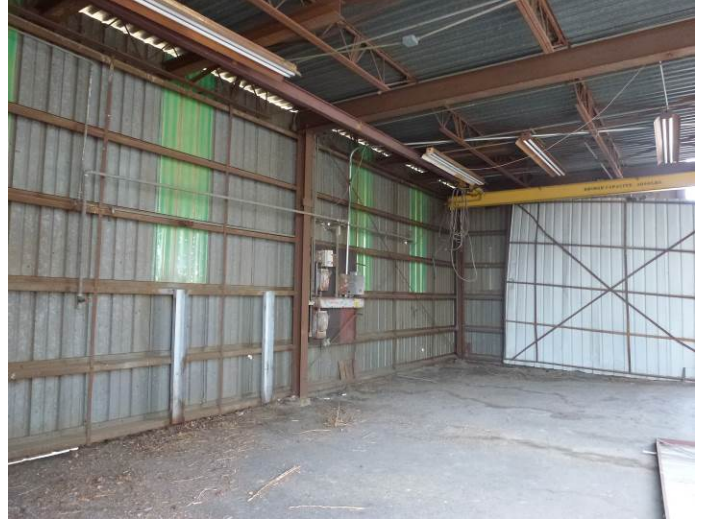
Image 14. Interior view of the Wash Building.
