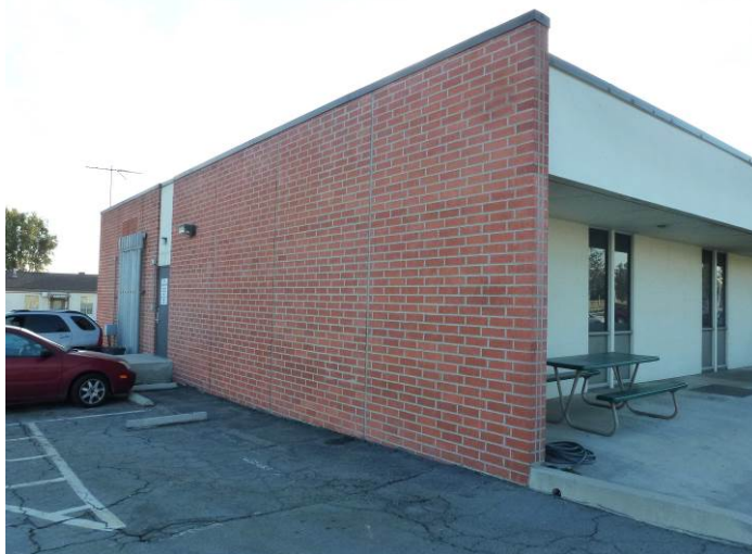
Image 3. View looking southwest at the east and north façades.
