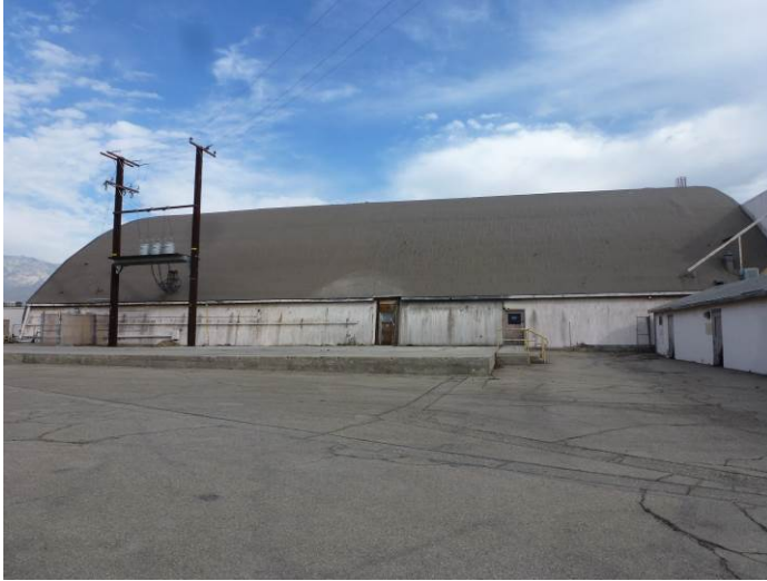
Image 1. View looking northeast at the southwest façade.
