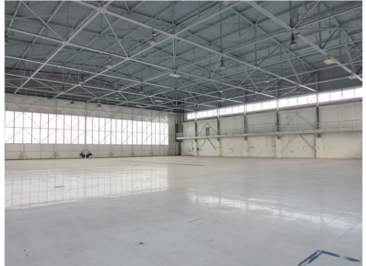
Image 10. Interior view of the hangar looking northeast.
