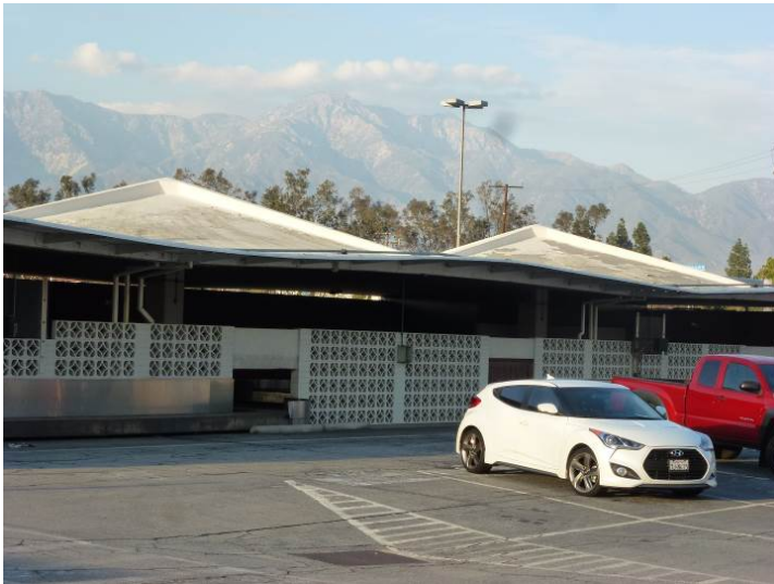
Image 13. View looking north at Baggage Claim Building B.
