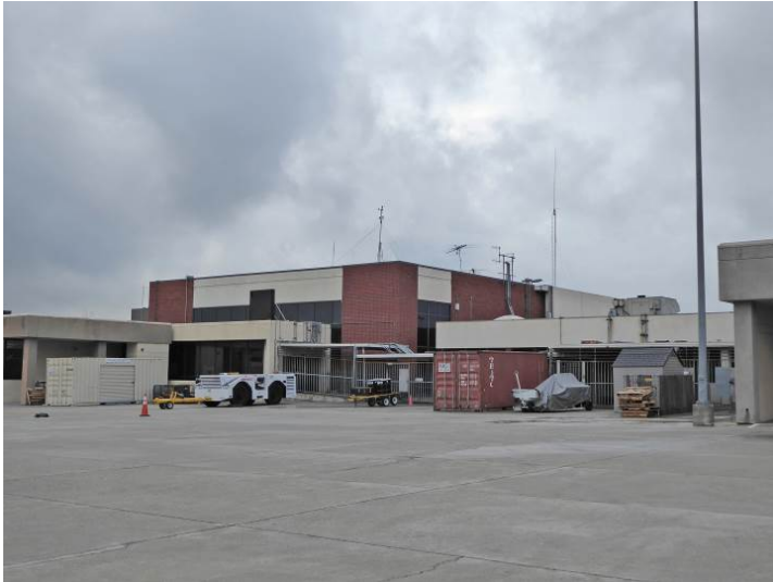
Image 17. View looking west from the runway area at the southeast and northeast façades of Terminal One.
