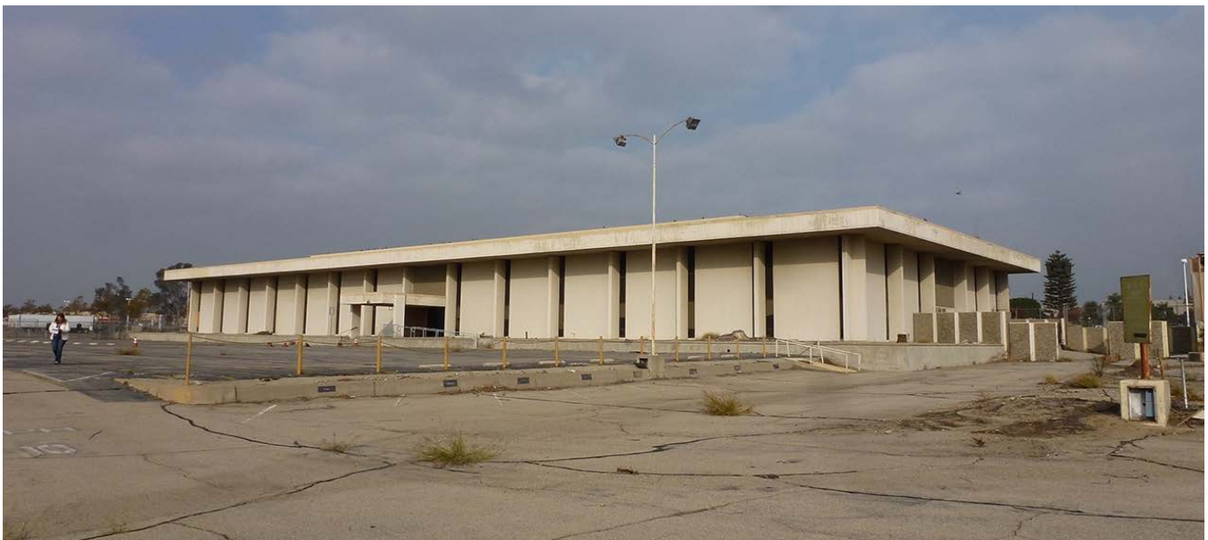
Below: Lockheed Administration Office Building No. 15
