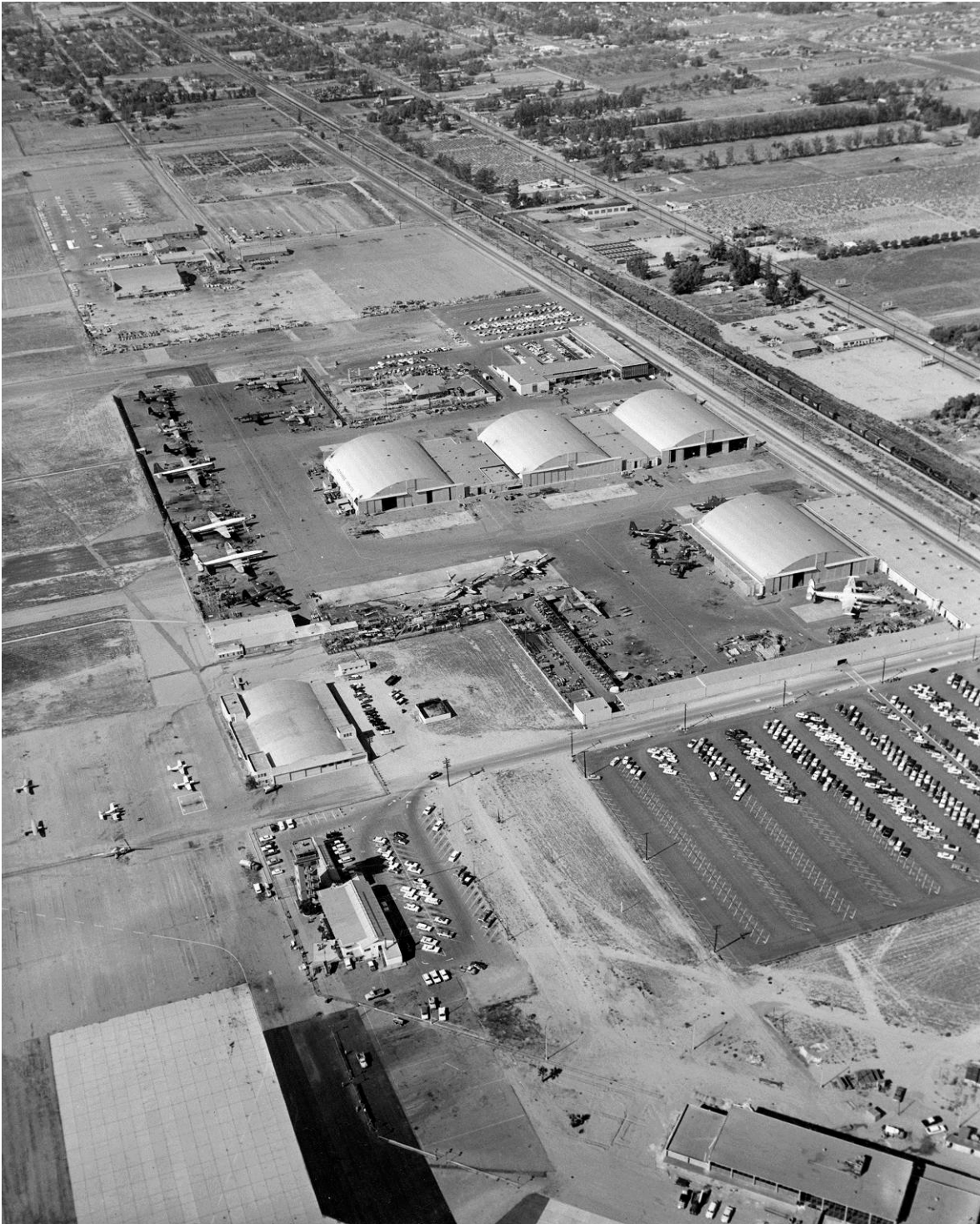
Image 7. Aerial view of LAS area (the hangar in the foreground right has been demolished), post-1953. Photographer: Gordon Ayers. Source: Ontario City Library Robert E. Ellingwood Model Colony Room. Accession No. 3677.
