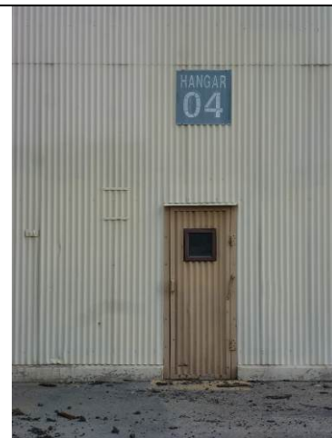
Image 6. Detail view looking east at west façade.
