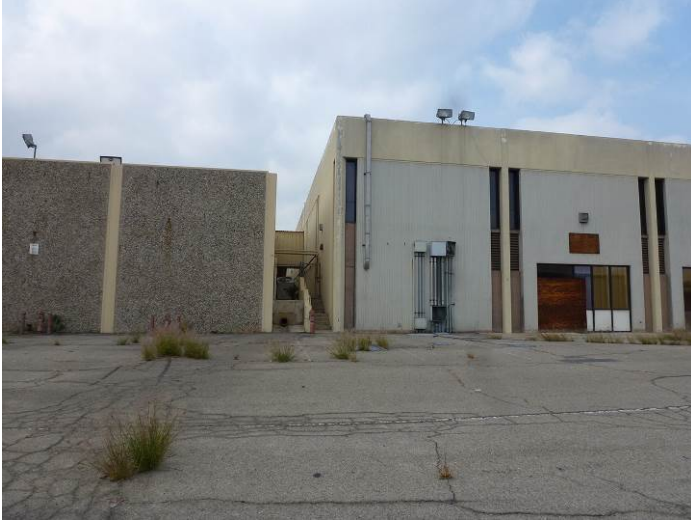
Image 1. View looking west at the east façade of Building 14 (left).
