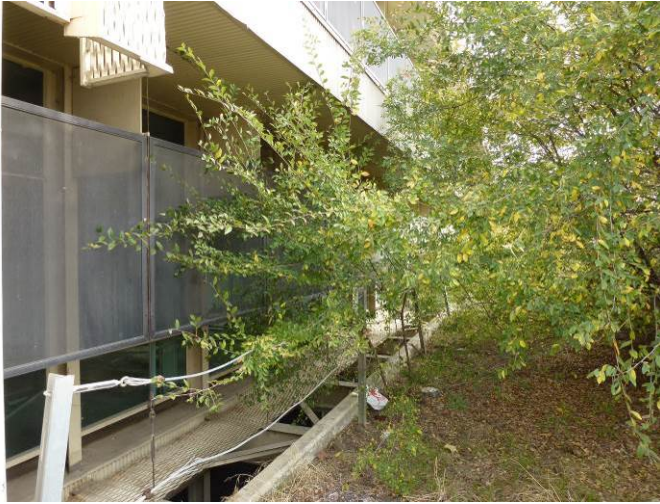
Image 5. Detail view looking northeast at the south façade.
