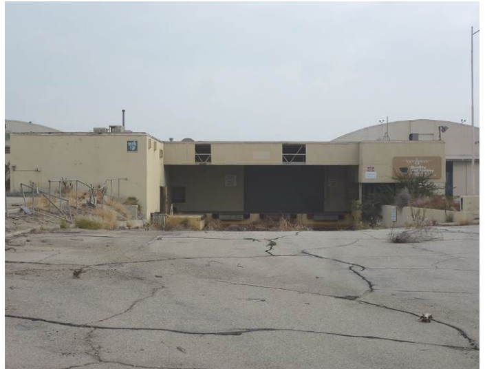
Image 2. View looking east at the west façade.
