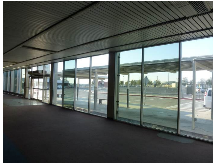
Image 4. Interior view looking west.
