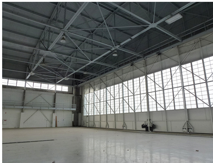
Image 11. Interior view of the hangar looking northwest.
