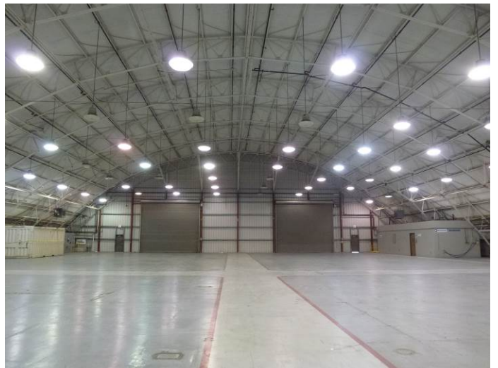
Image 4. Interior view looking southeast.
