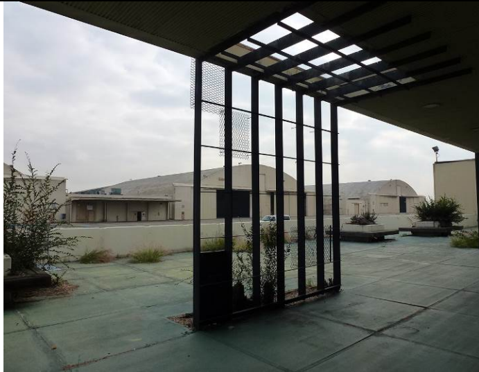
Image 3. Detail view looking southeast from Building 11.
