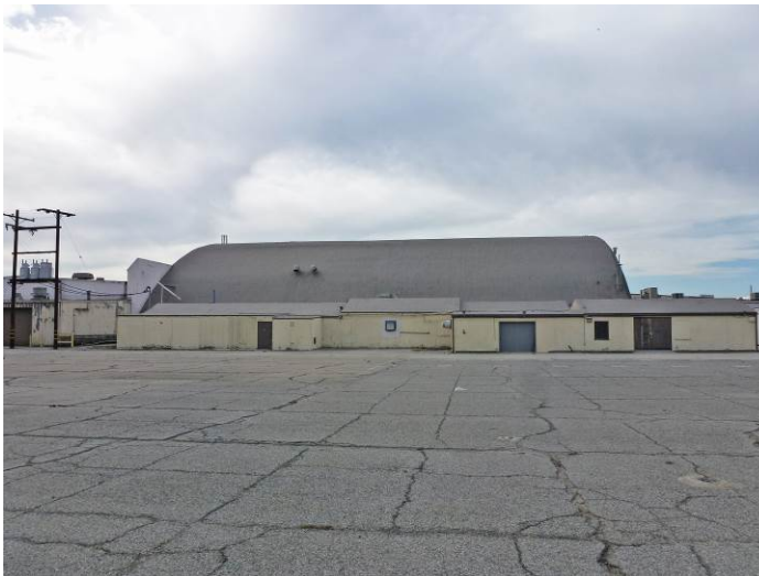
Image 3. View looking southwest at the northeast façades of Building M and Hangar 4.
