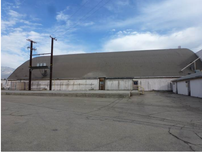
Image 1. View looking northeast at the southwest façade.
