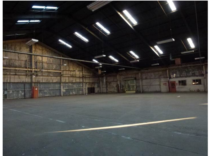
Image 4. Interior view looking southeast.
