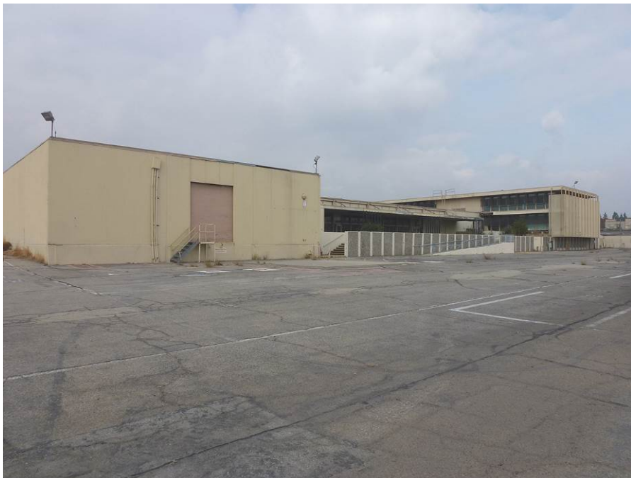
Image 2. View looking northwest at the east façades of the Mail Room, the Cafeteria, and the Executive Office Building.
