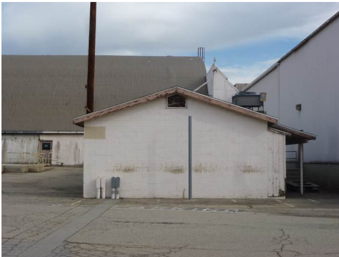
Image 7. View looking northeast at the southwest façade of Building J.
