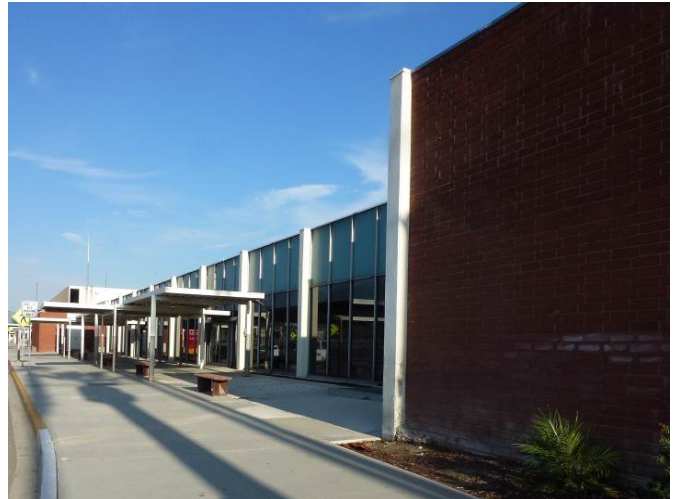
Image 2. View of Terminal One primary facade looking east. The historic core of the Terminal One building is recommended as a contributor to the historic district.
