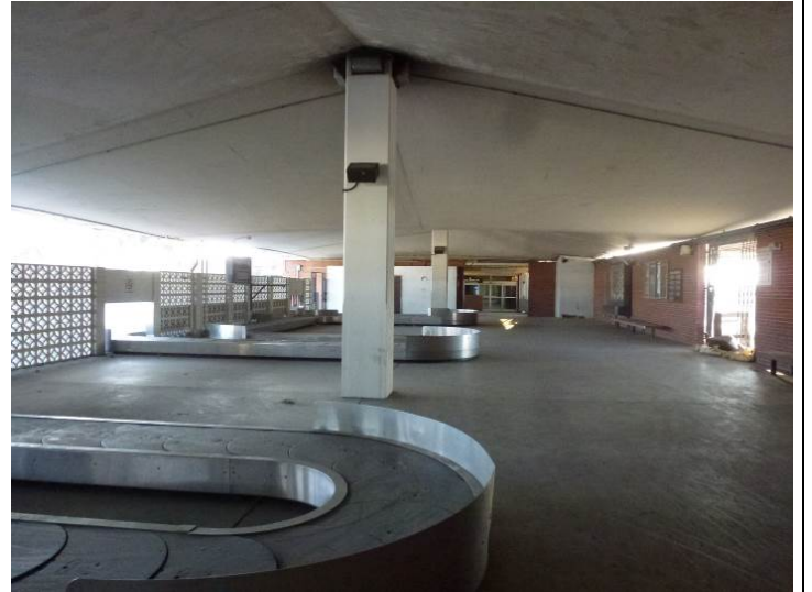
Image 4. Interior view looking west.
