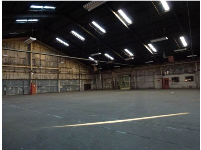
Image 4. Interior view looking southeast.
