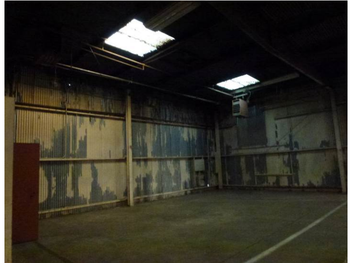
Image 6. Interior view of south wing.
