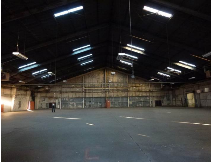
Image 5. Interior view looking southwest.
