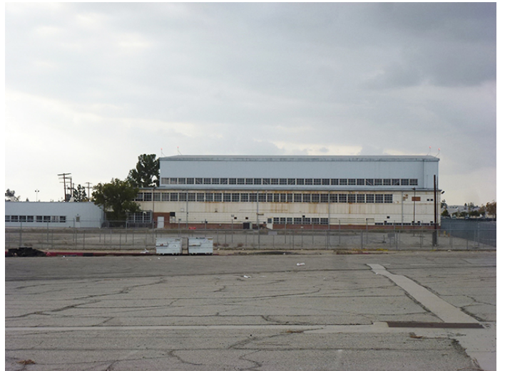
Image 8. View looking west at the east façade.
