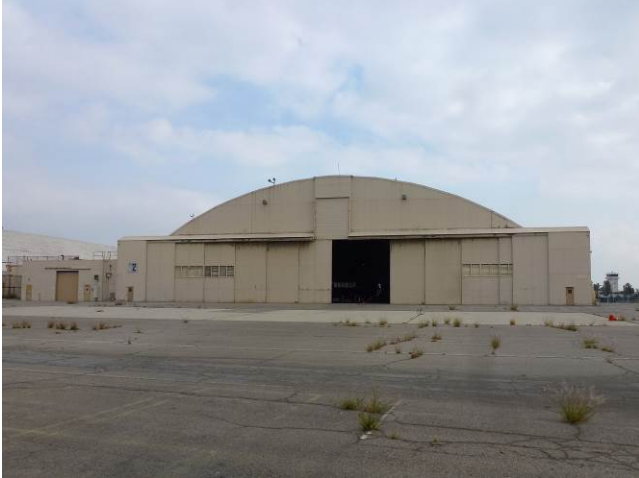
Image 1. View looking north at the south façade.
