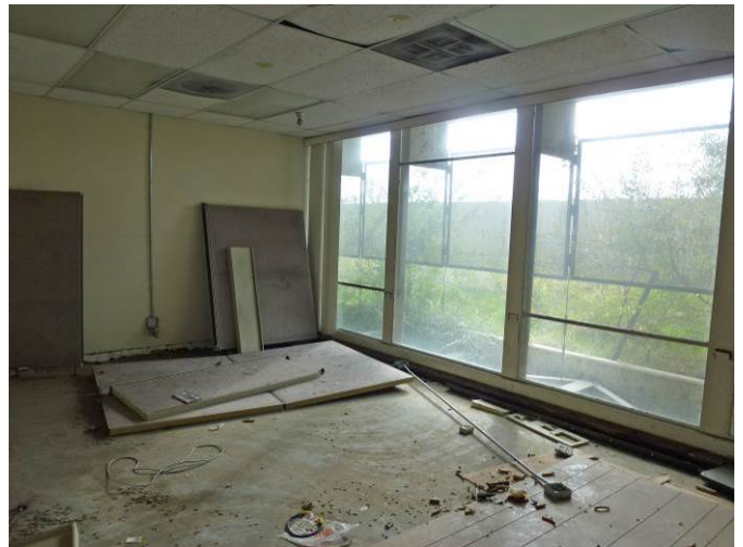
Image 8. View of the first-floor interior looking southeast.
