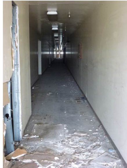
Image 4. View of the interior looking west.
