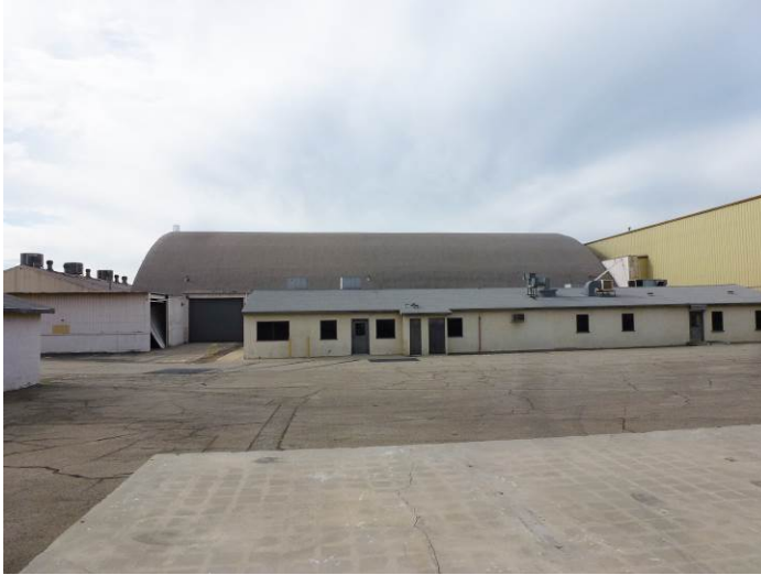
Image 1. View looking southwest at the northeast façades of Hangar 3 and the Commissary Building.
