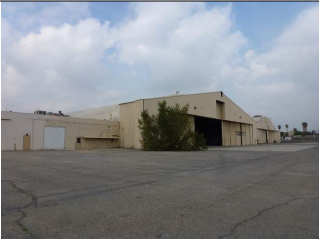
Image 3. View looking northwest at the east façade.
