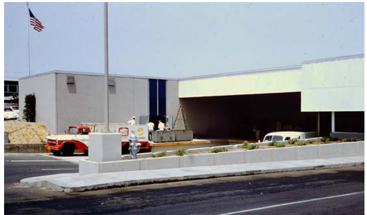
Image 4. View looking northeast at the west and south façades, ca. 1956. Source: Collection of Colin Russell.
