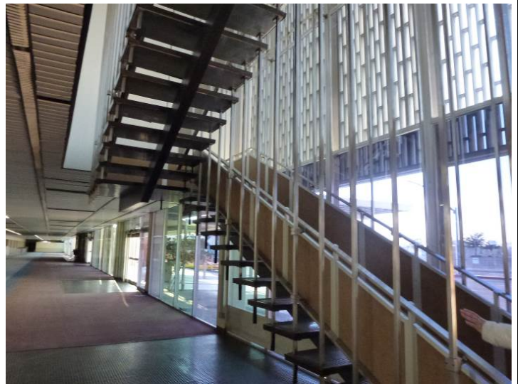
Image 8. Interior view looking southwest.
