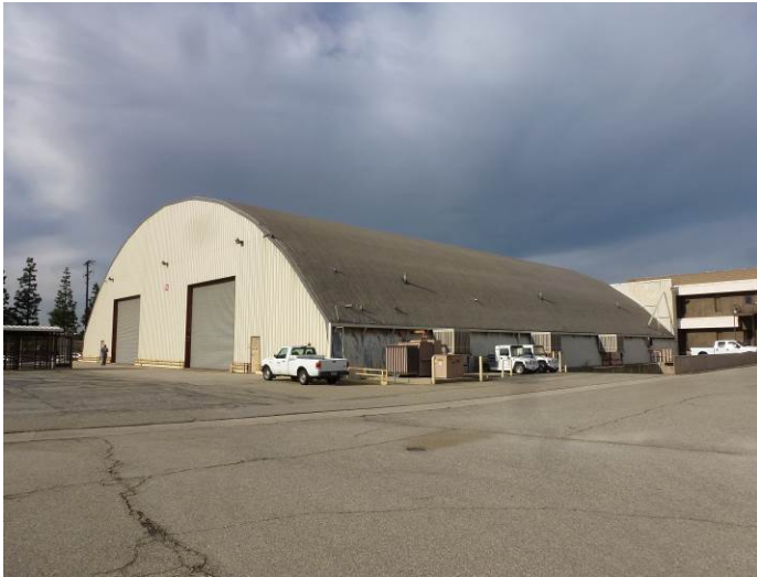
Image 1. View looking north at the southeast and northeast façades.
