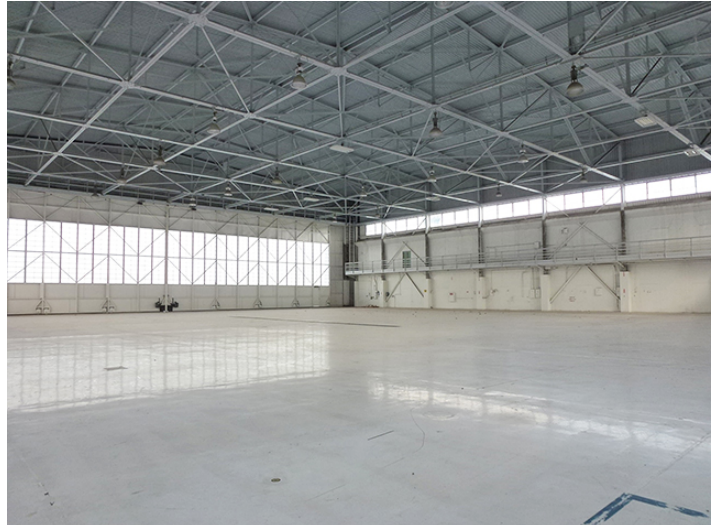
Image 10. Interior view of the hangar looking northeast.
