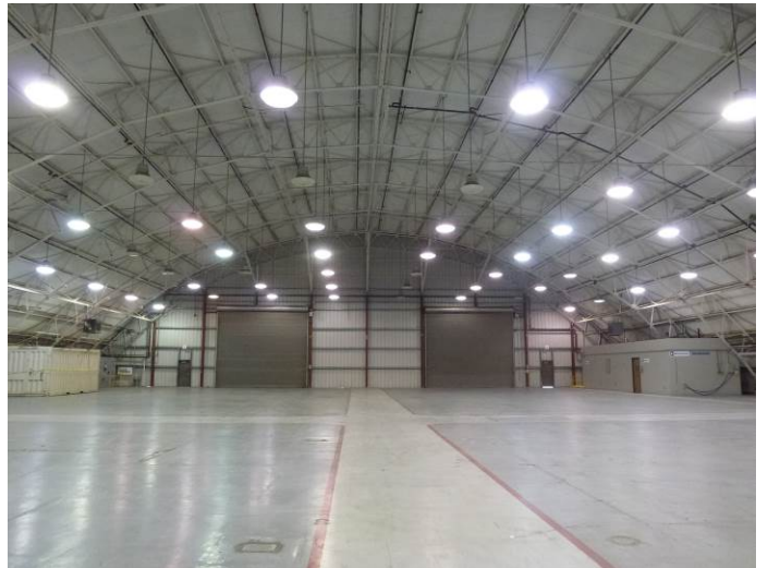
Image 4. Interior view looking southeast.
