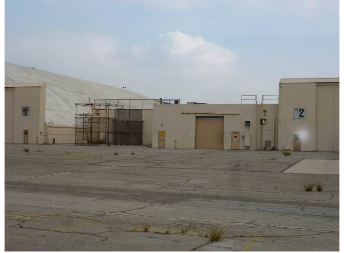
Image 2. View looking east at the west façade.
