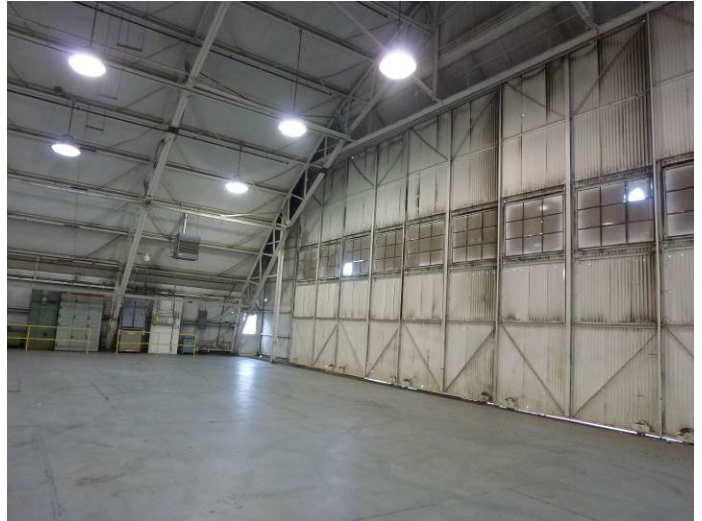
Image 6. Detail view of the interior looking west.
