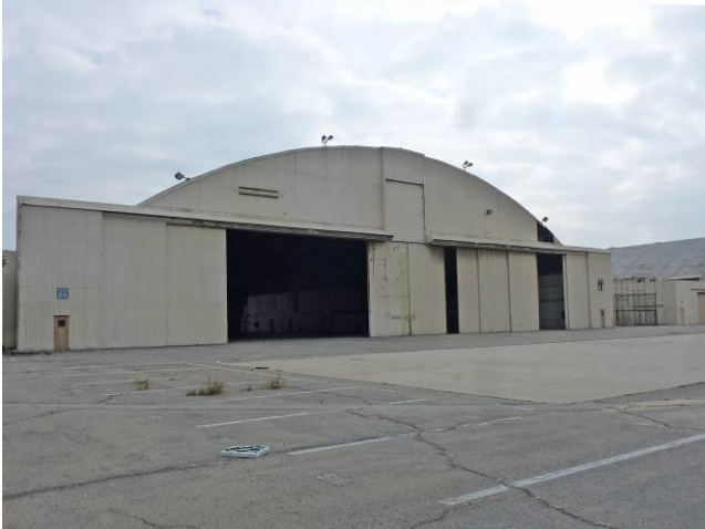
Image 1. View looking southeast at the west façade.
