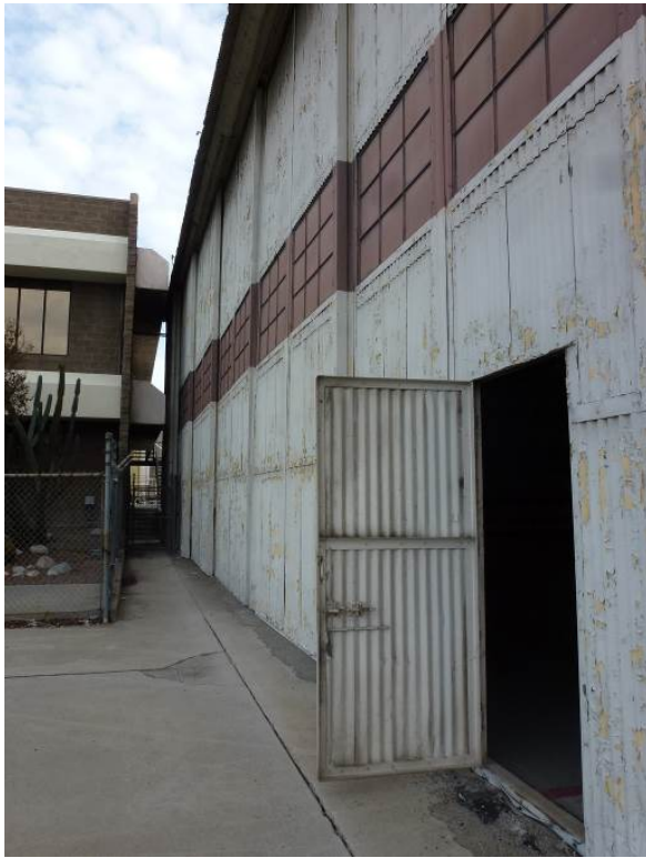
Image 3. Detail view looking at the northwest façade.
