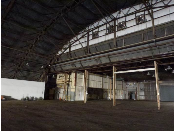
Image 5. Detail interior view looking east.
