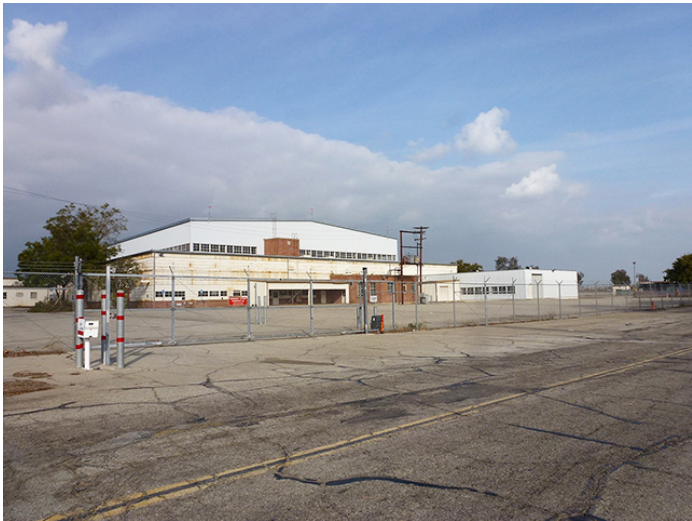
Image 7. View looking northeast at the west and south façades.
