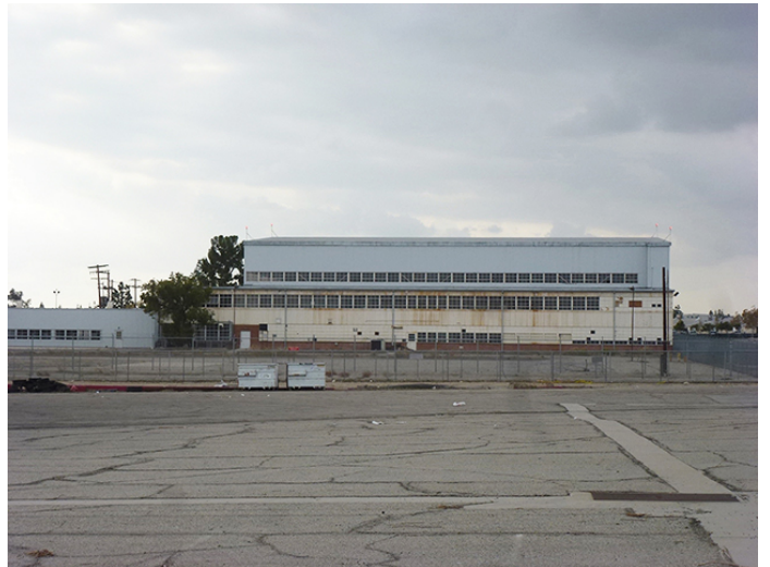
Image 8. View looking west at the east façade.
