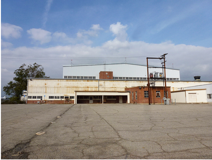
Image 5. View looking north at the south façade.
