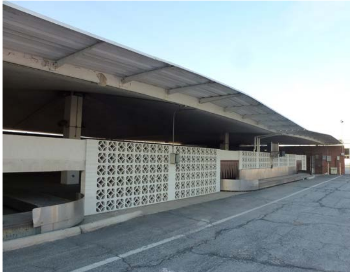
Image 3. Detail view looking north at the southwest façade.
