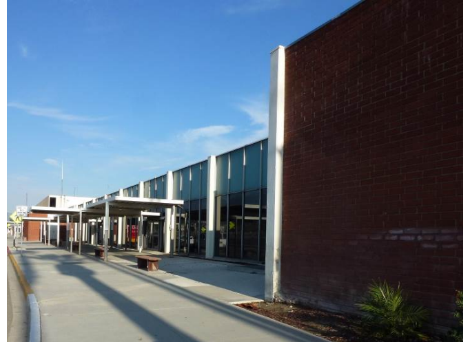
Image 2. View of Terminal One primary facade looking east. The historic core of the Terminal One building is recommended as a contributor to the historic district.
