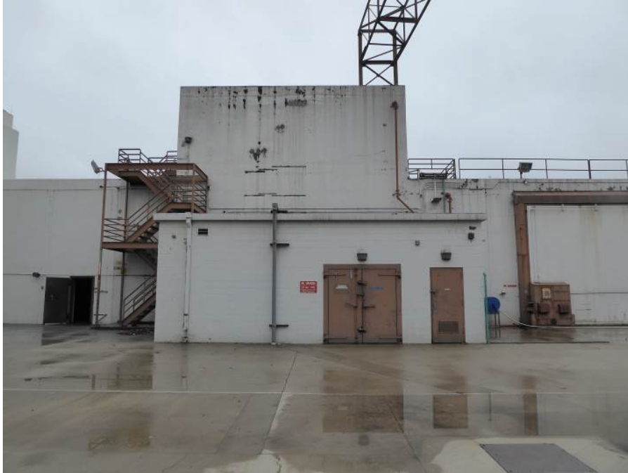
Image 5. View looking east at the Jet Engine Test Cell area. ASM, December 1, 2016.
