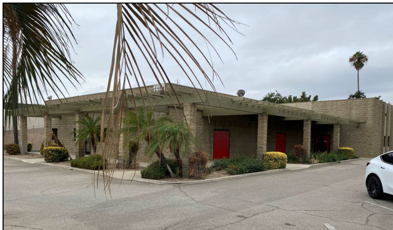
Northeast portion of Project Site facing southwest
