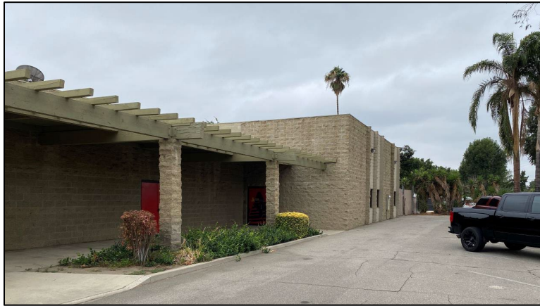
Northern Elevation of Project Site facing west
