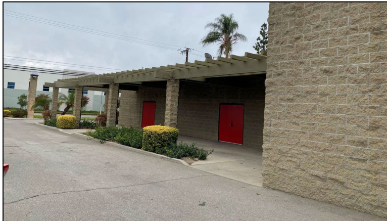
Northern Elevation of Project Site facing east
