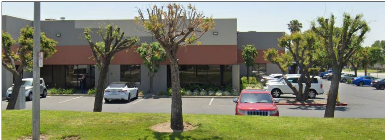
North elevation of project suite (Units 106 and 107) facing Locust Street.
