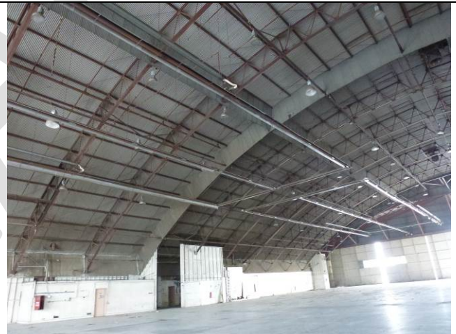
Image 4. Interior view looking northeast.
