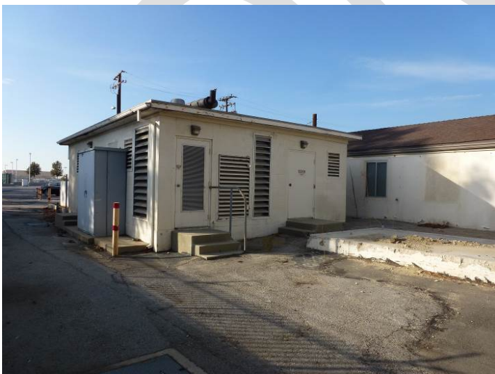
Image 11. View looking northwest at the south and east façades of ancillary building to the west of the control tower.
