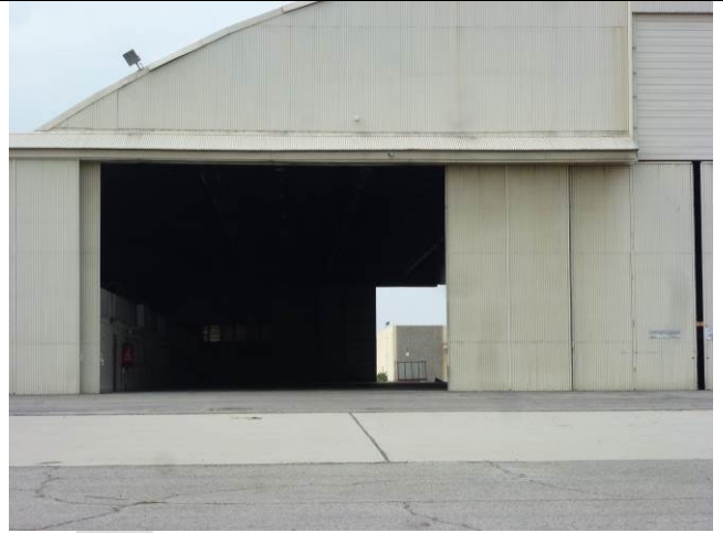
Image 6. Detail view looking west at the south façade.
