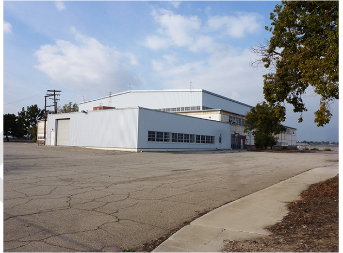
Image 6. View looking northwest at the south and east façades.
