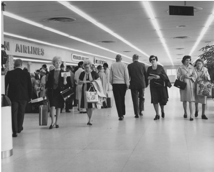
Image 25. Historic view of the ticketing hall. January 1968.
