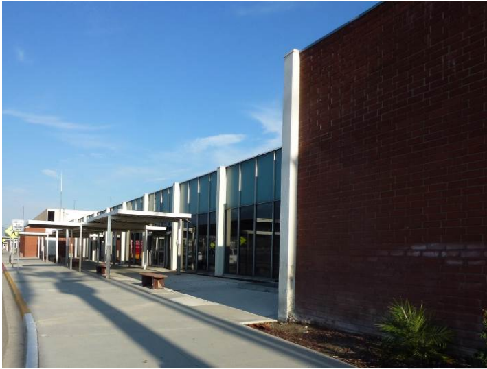
Image 1. Detail view looking east at the northwest façade.
