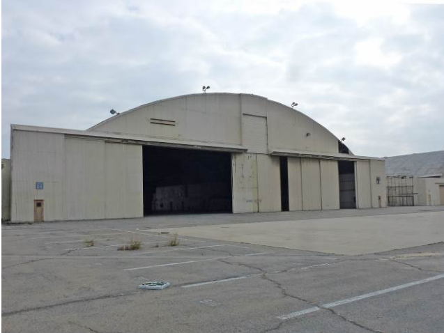
Image 1. View looking southeast at the west façade.
