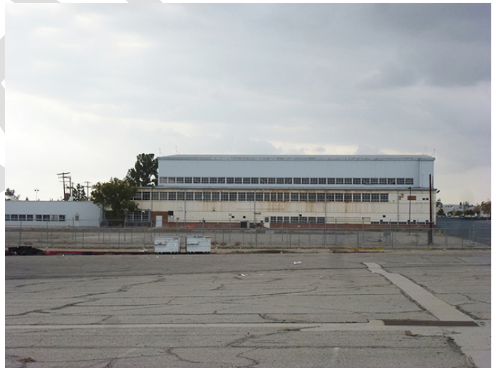
Image 8. View looking west at the east façade.
