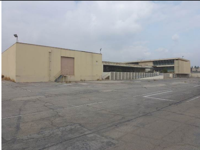
Image 1. View looking northwest at the west and east façades of buildings 12, 11, and 10.
