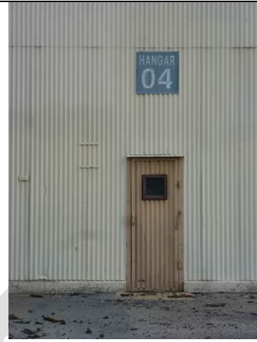
Image 6. Detail view looking east at west façade.
