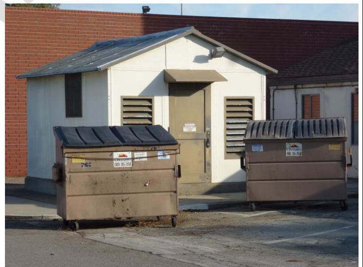
Image 12. View looking southeast at north and west façades of ancillary building to the north of the control tower.
