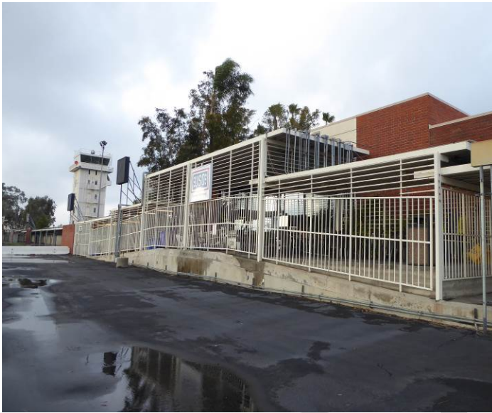
Image 5. View of Control Tower looking west from runway.
