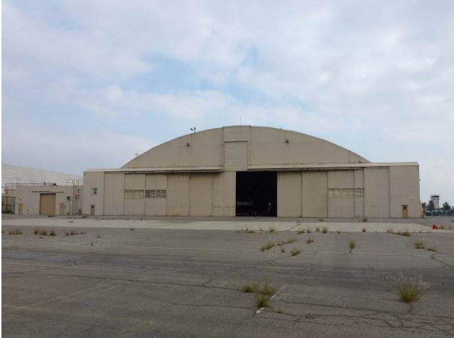
Image 1. View looking north at the south façade.
