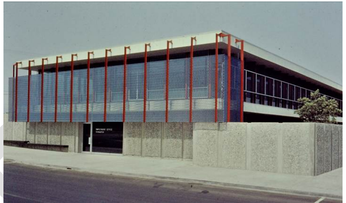
Image 10. View looking northeast at the west and south façades, ca. 1956. Source: Collection of Colin Russell.
