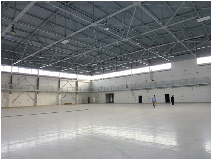
Image 13. Interior view of the hangar looking southeast.
