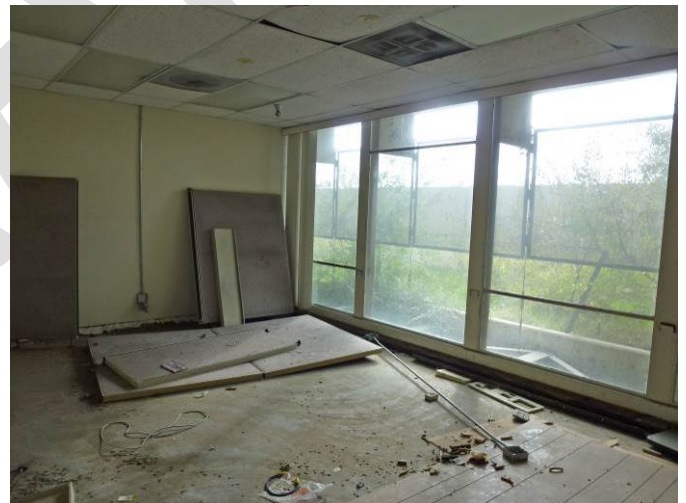
Image 8. View of the first-floor interior looking southeast.
