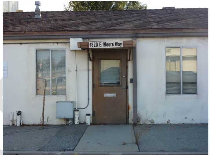
Image 10. View looking south at the north façade of ancillary building north of the control tower.
