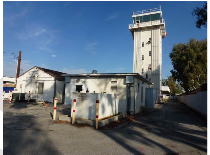
Image 18. View looking northeast at the west façades of the Control Tower and ancillary buildings.
