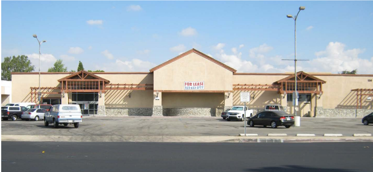
View looking north from G Street Subject Building)
