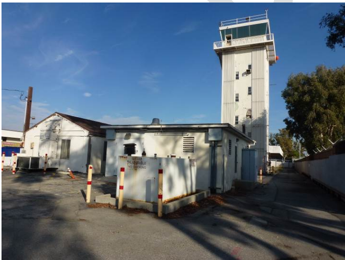
Image 3. View of Control Tower and ancillary buildings looking east.
