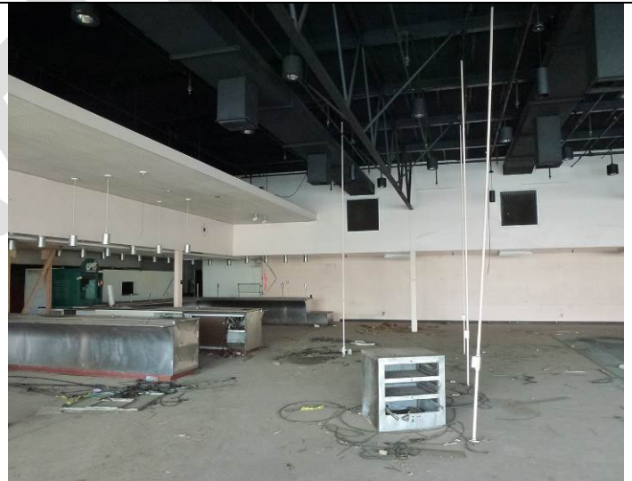
Image 4. Interior view looking southwest.
