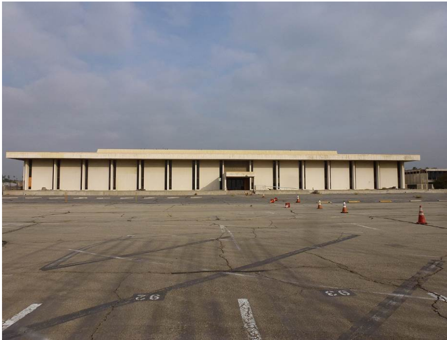
Image 1. View looking north at the south façade of Building 15.
