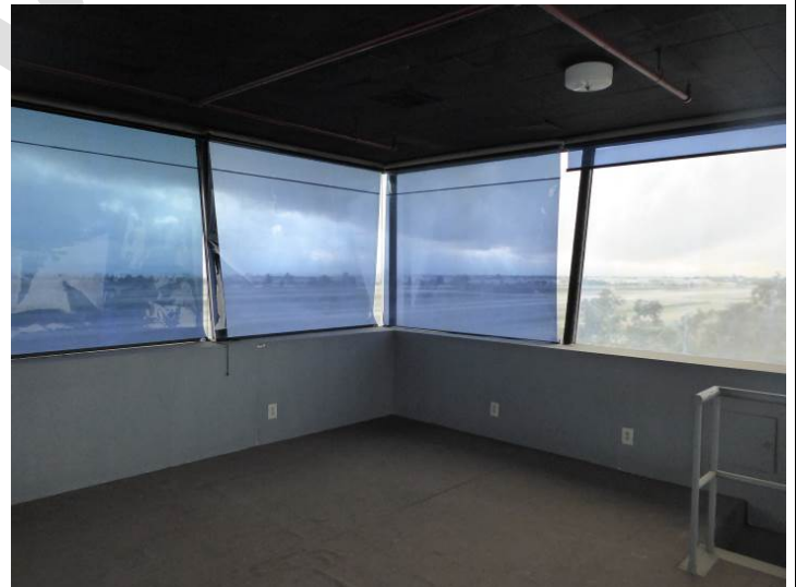
Image 8. Interior view of the control room looking southwest.
