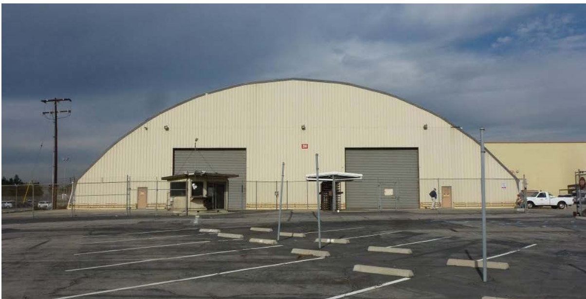
Below: GE Hangar 7
