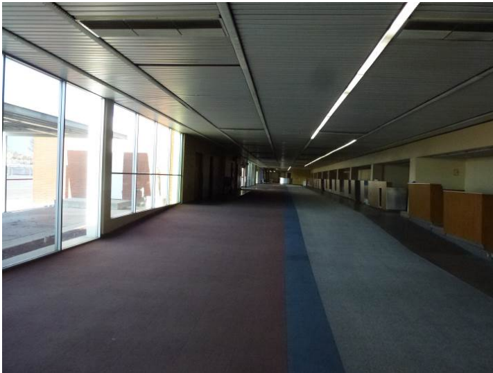
Image 5. Interior view of ticketing area looking northeast.
