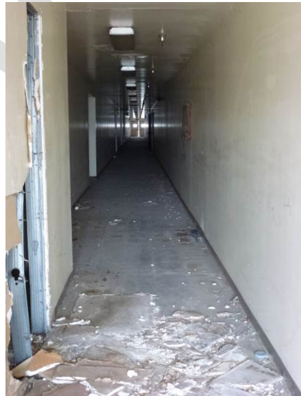
Image 4. View of the interior looking west.
