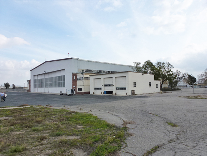
Image 1. View looking southeast at the north and west façades, with Fire Station in the foreground.
