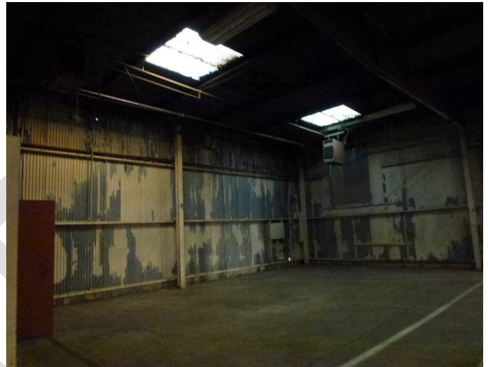
Image 6. Interior view of south wing.
