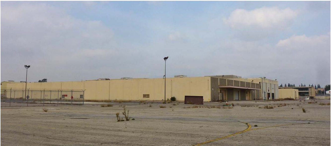
Above: Lockheed Warehouse, Building No. 14
