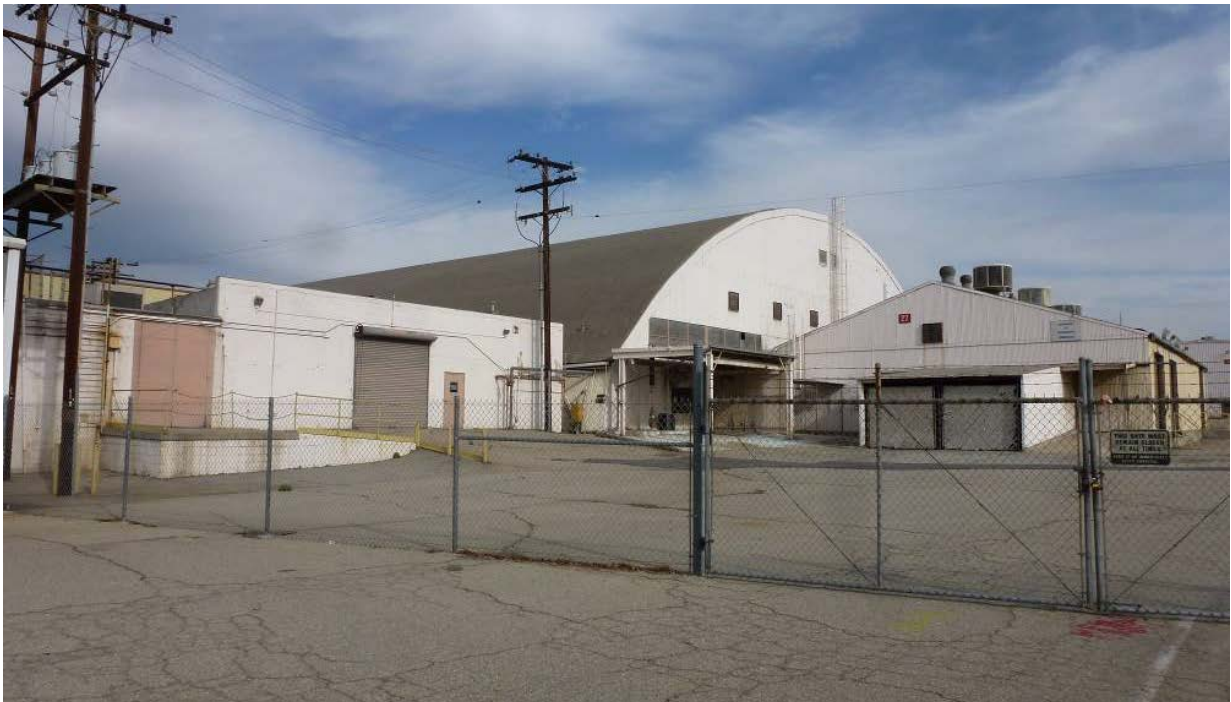
Below: GE Hangar 4
