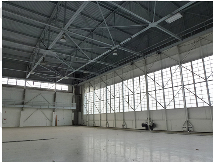
Image 11. Interior view of the hangar looking northwest.
