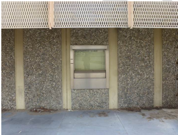
Image 3. Detail view looking east at the west façade.
