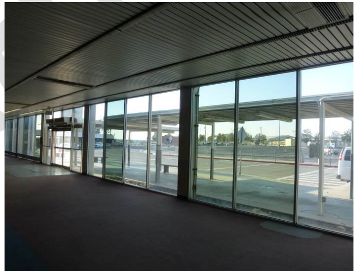
Image 4. Interior view looking west.
