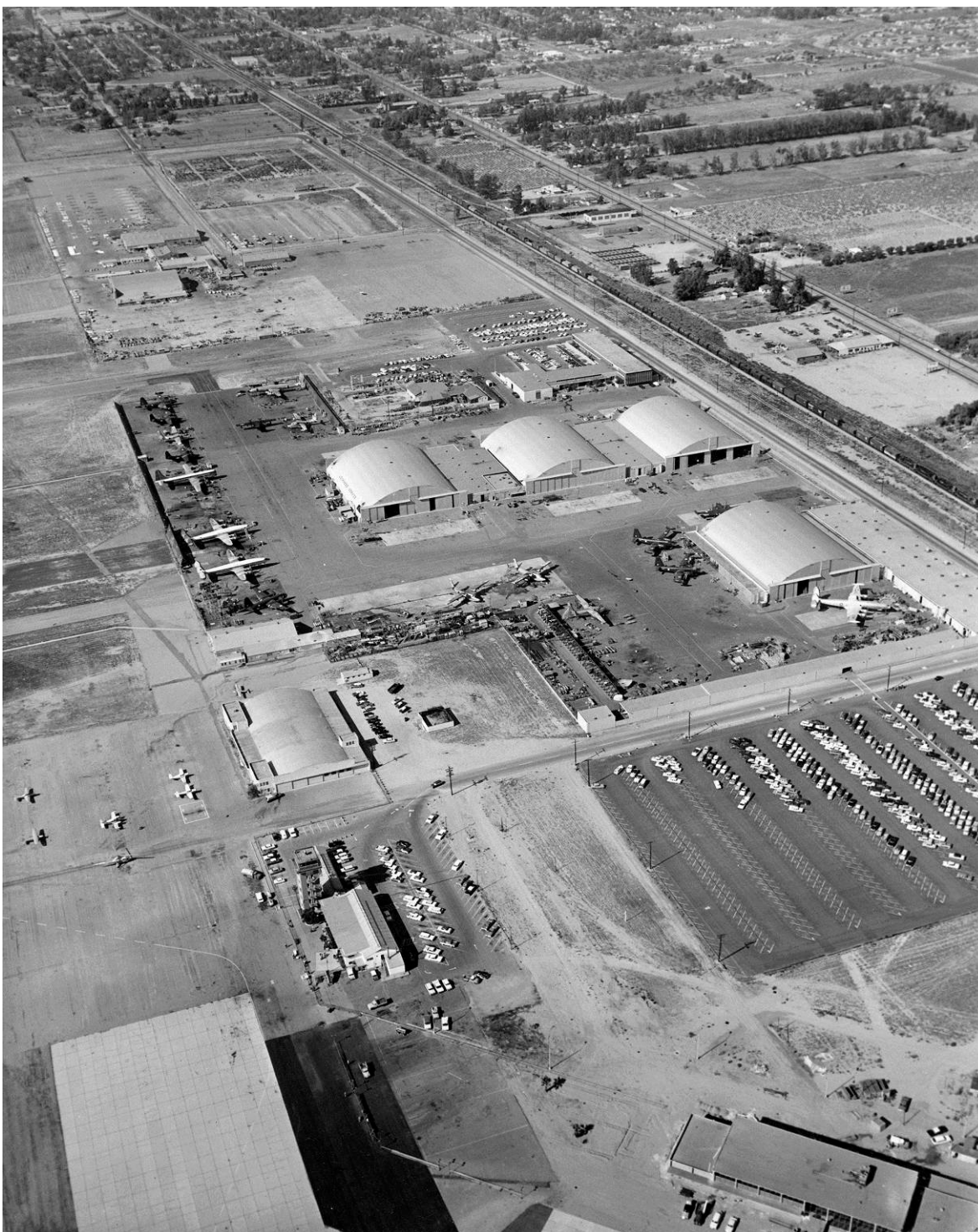
Image 7. Aerial view of LAS area (the hangar in the foreground right has been demolished), post-1953. Photographer: Gordon Ayers. Source: Ontario City Library Robert E. Ellingwood Model Colony Room. Accession No. 3677.
