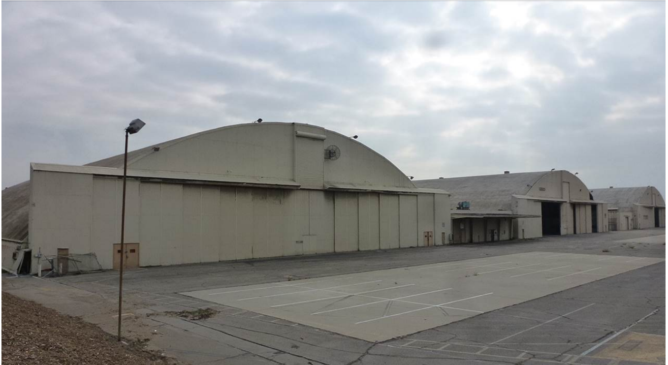
Above: (Left to right) Lockheed Hangar 6, Building No. 5, Lockheed Hangar 4 Warehouse, Building No.3, and Lockheed Hangar 2
