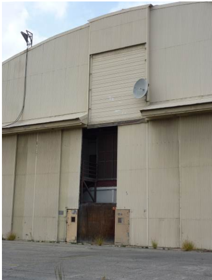
Image 3. Detail view looking southwest at the east façade.
