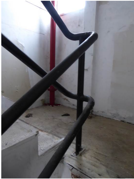
Image 5. Detail view of the interior staircase.
