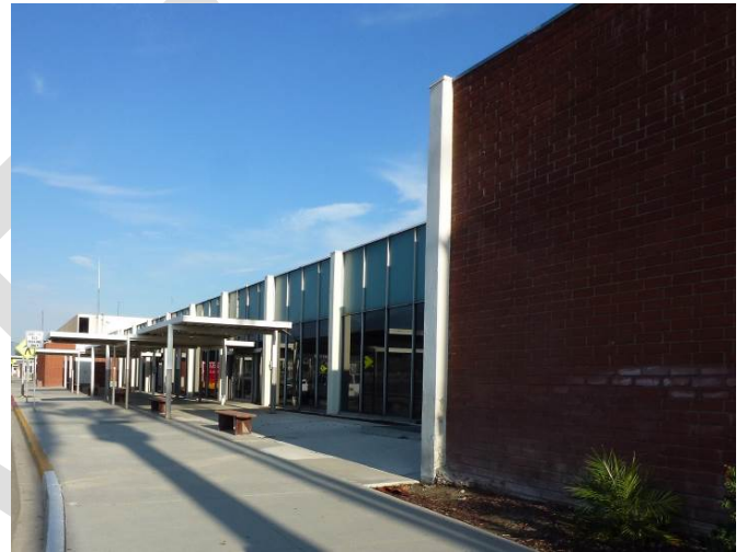
Image 2. View of Terminal One primary facade looking east.
