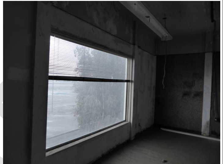
Image 6. Interior view looking southwest of an office in the Control Tower.
