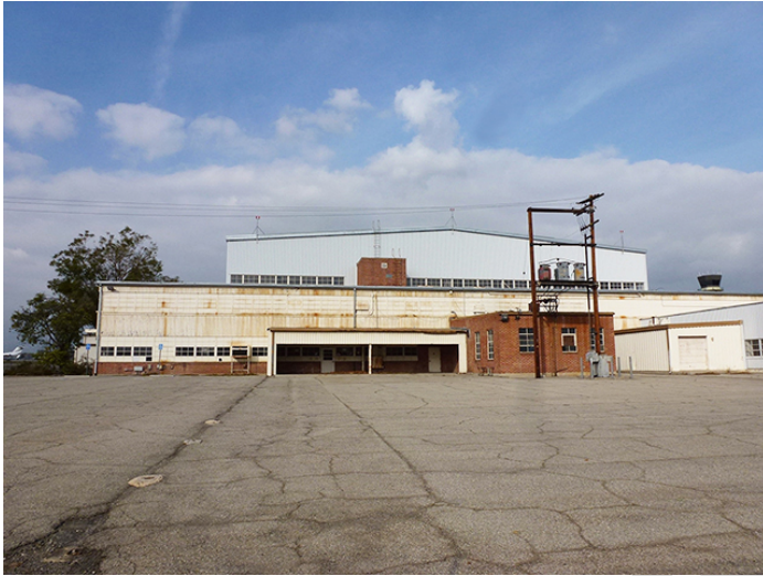
Image 5. View looking north at the south façade.
