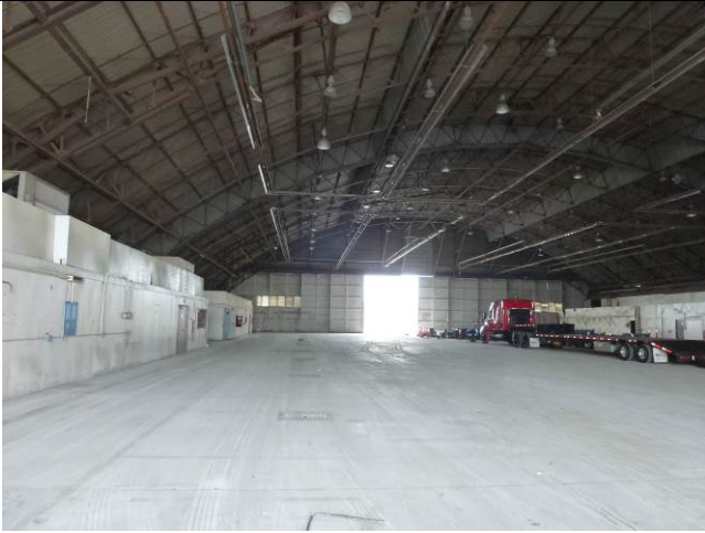
Image 5. View of the interior looking west.
