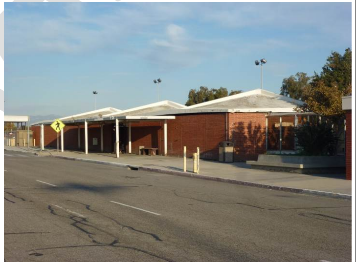
Image 12. View looking east at the northwest and southwest façades of Baggage Claim Building B.
