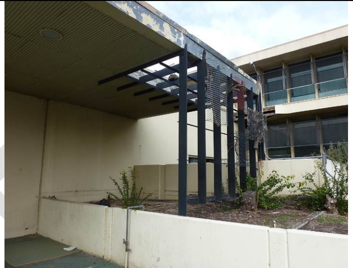
Image 2. Detail view looking northwest at the east façade of Building 11 and the south façade of Building 10.
