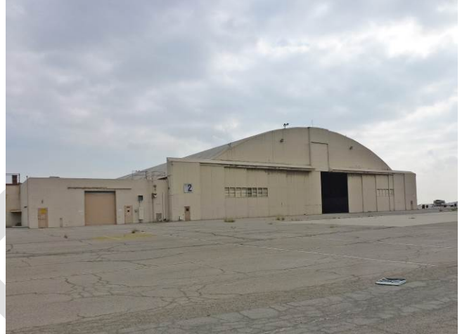
Image 2. View looking southeast at the north and west façades.
