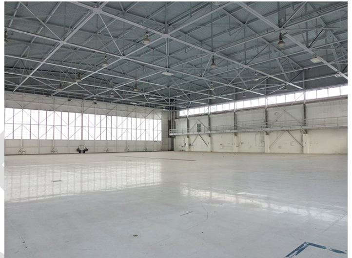
Image 10. Interior view of the hangar looking northeast.
