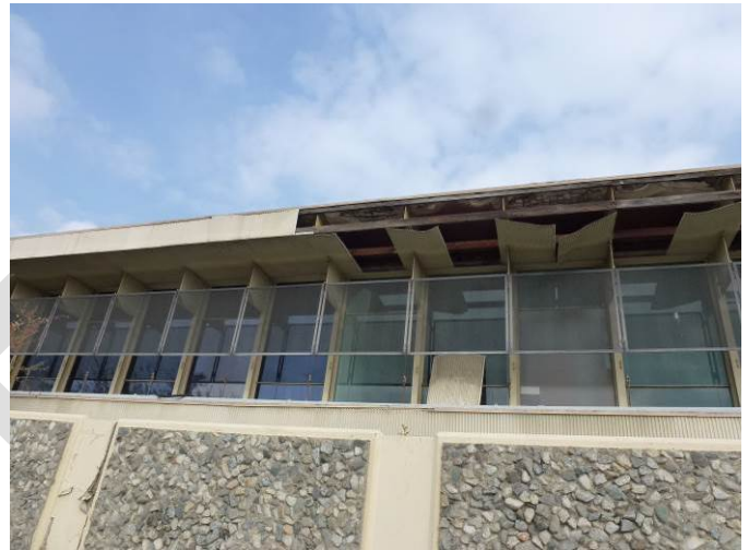
Image 6. Detail view of the south façade.
