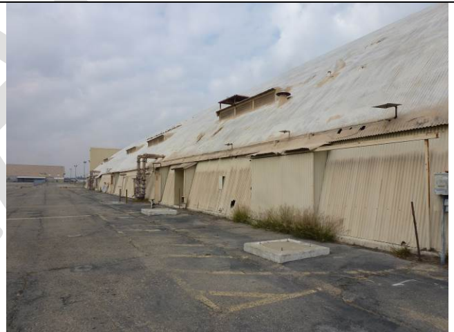
Image 4. Detail view looking northwest at the south façade.
