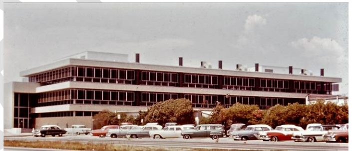
Image 12. View looking northeast at the west and south façades, ca. 1956. Source: Collection of Colin Russell.
