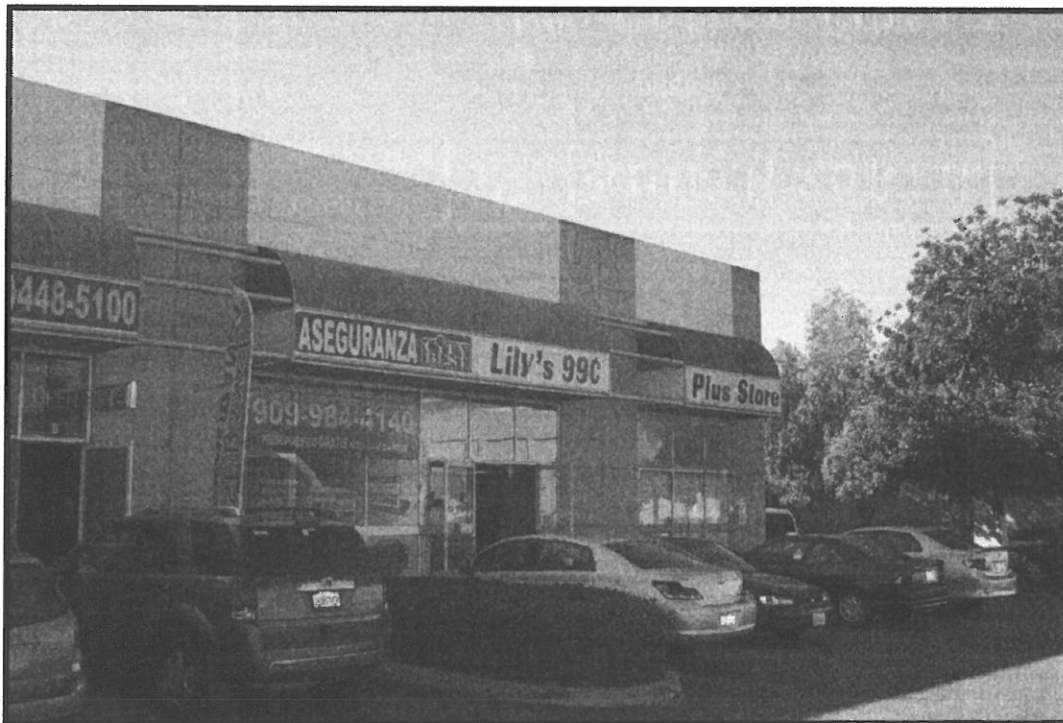
New Store Frontage (Tenant Space "AB")
