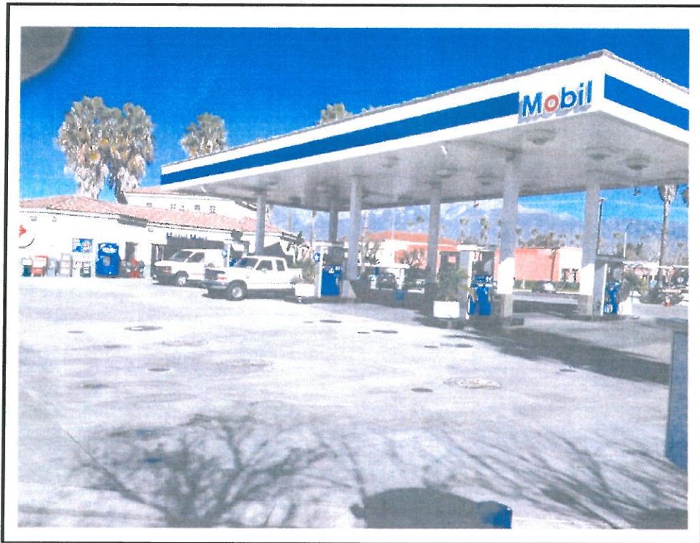
Exterior – Fueling Canopy
