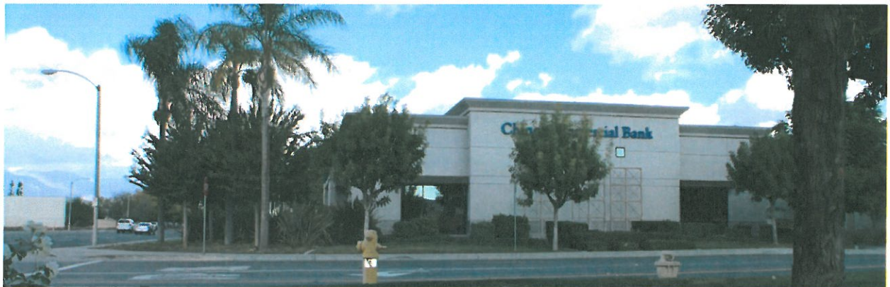
Above: North of Project Site
