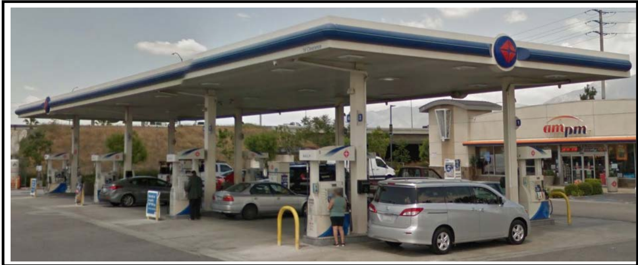
Arco Service Station and AM/PM Store – Looking North
