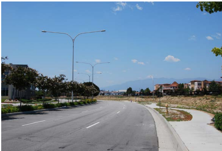
Views of streetscape along Concours Street at western portion
