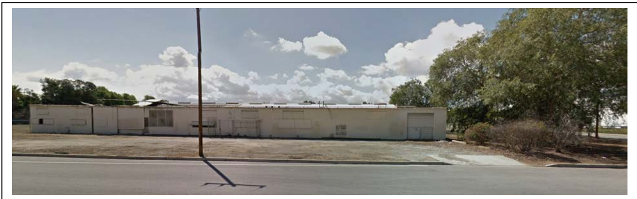
1431 South Baker Avenue – Acacia Street Frontage (Corner Lot): Looking South
