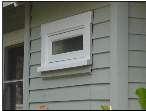
Example of an appropriate window alteration
