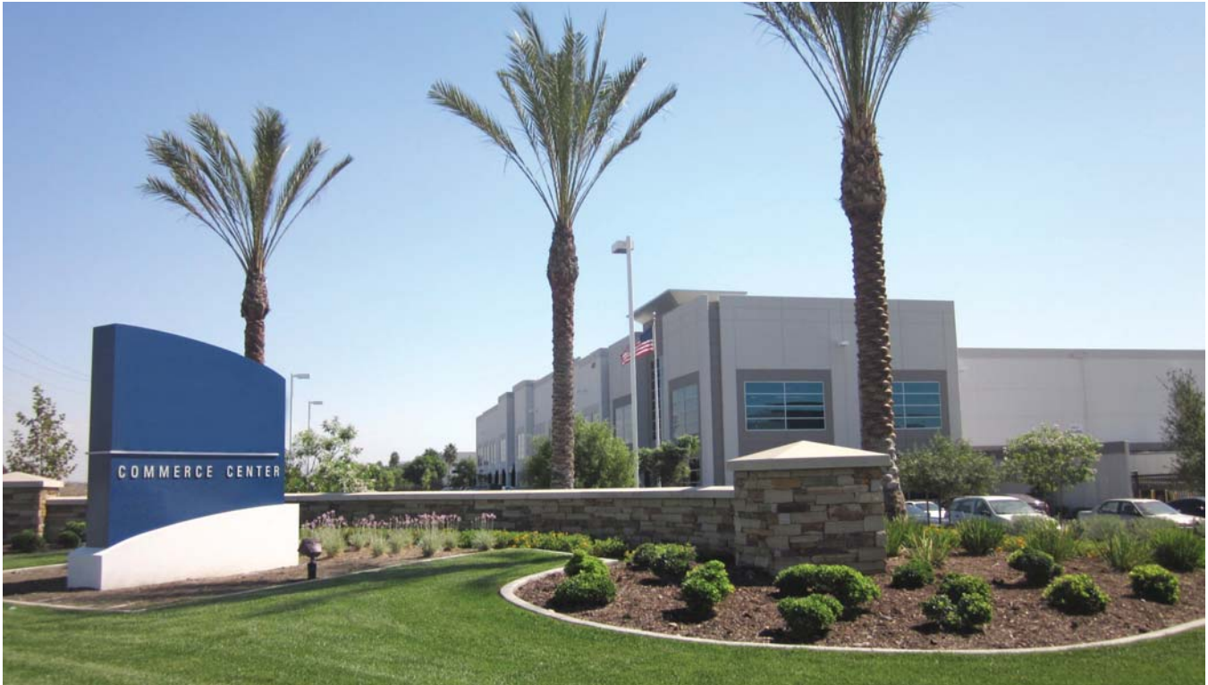
Photo 7.3 - Example of Industrial building
