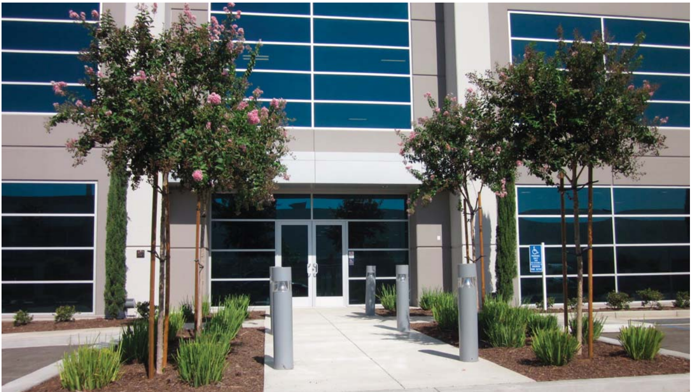
Photo 7.5 - Example of Industrial lighting at office entry
