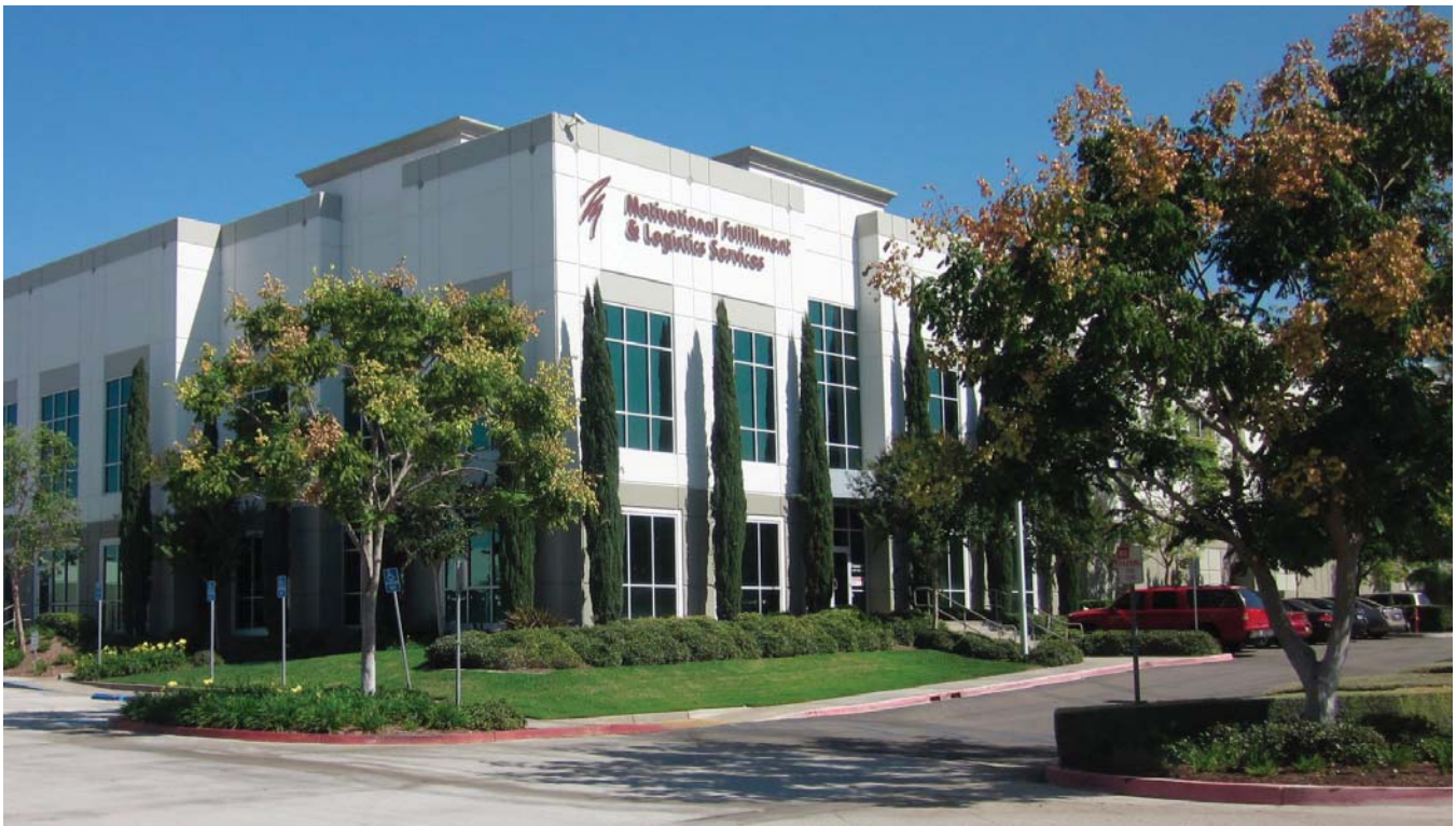
Photo 7.2 - Example of Industrial building
