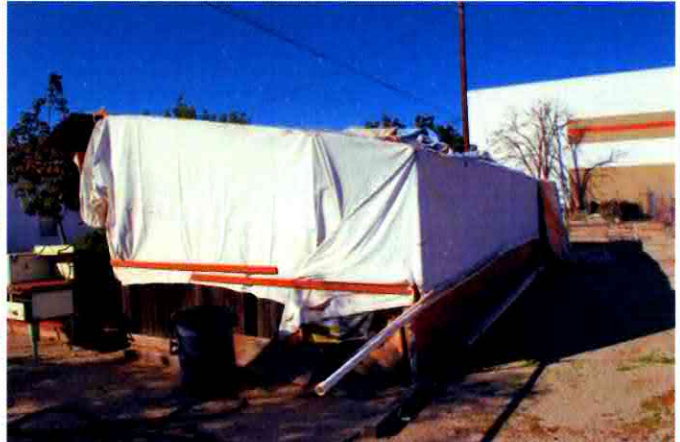
Chicken Coop: North and east elevations, view southwest
