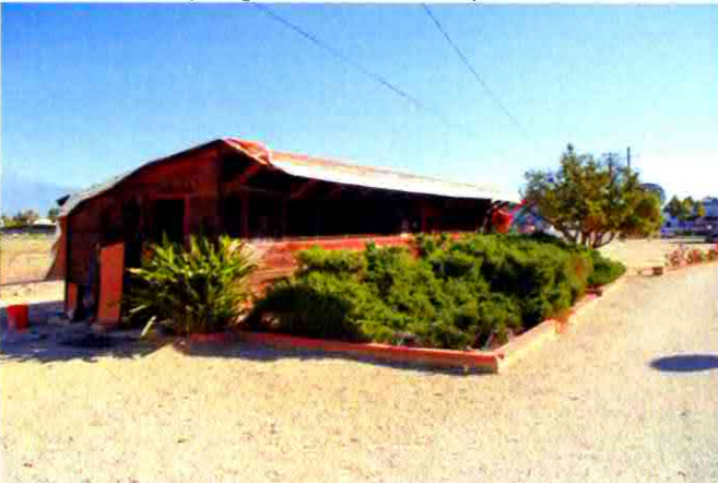
Chicken Coop: South and west elevations, view northeast
