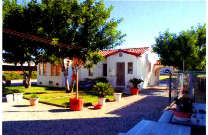
West and south elevation, view northeast
