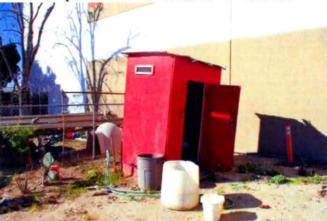
Privy: North and east elevations, view southwest
