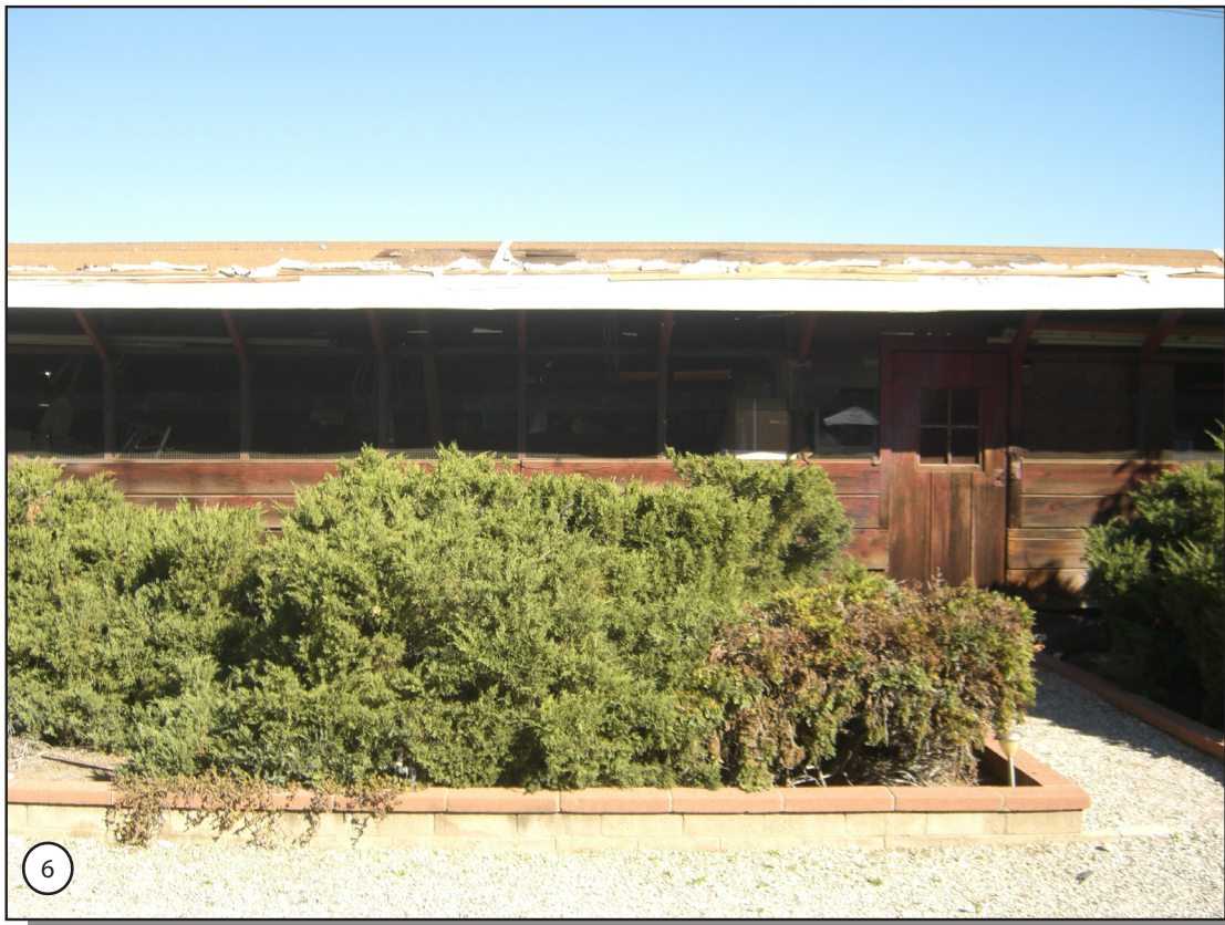
Photograph 6: Chicken Coop, View towards the north.
