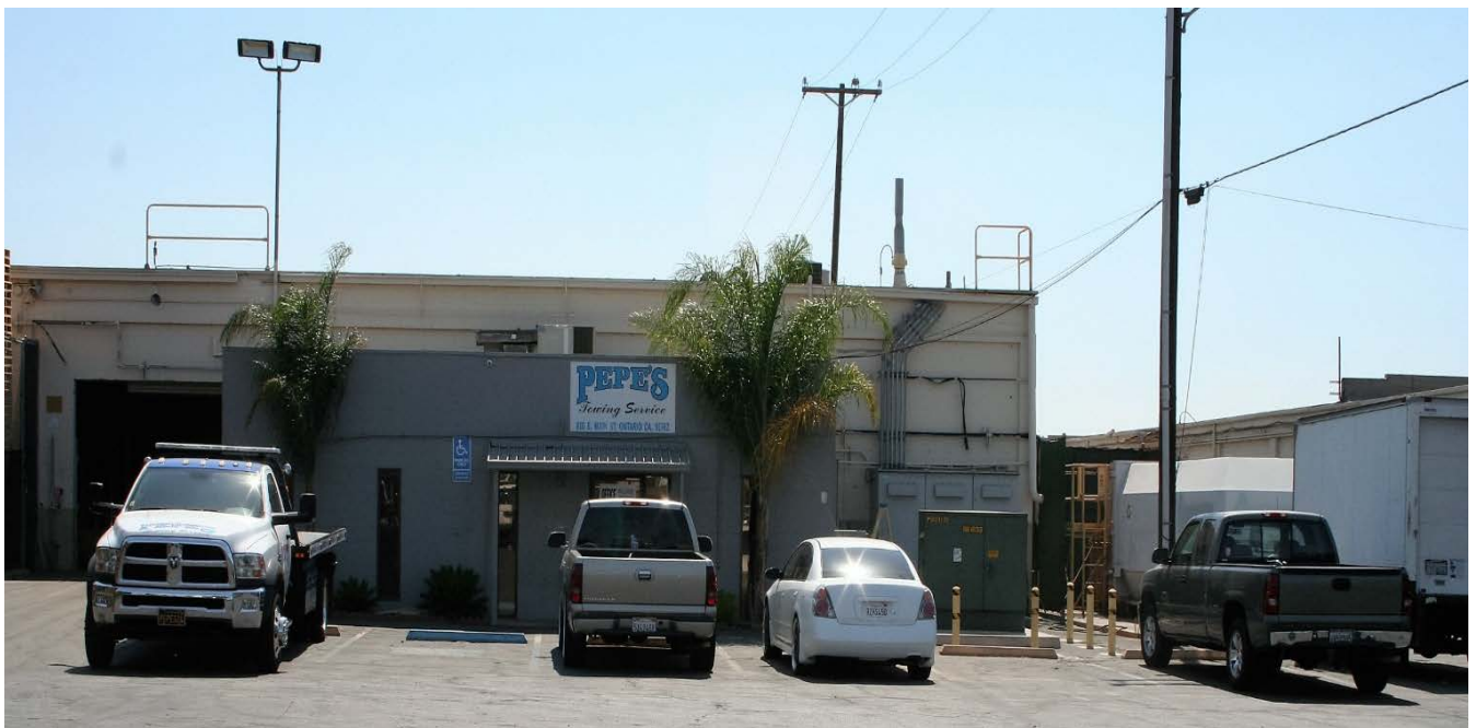
View Looking East at Front of Pepe's Towing Service Office (Building 2)
