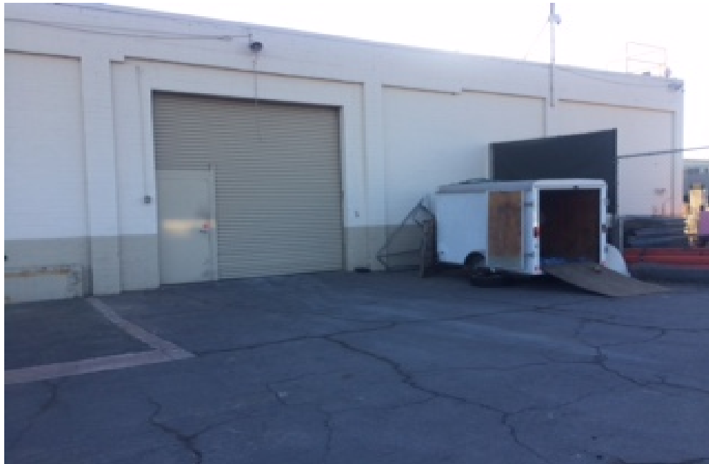
View Looking East at Vehicle Evidence Room
