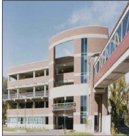
An example of a pedestrian bridge between buildings. Use of glass allows for visibility while protecting pedestrians from the elements.
