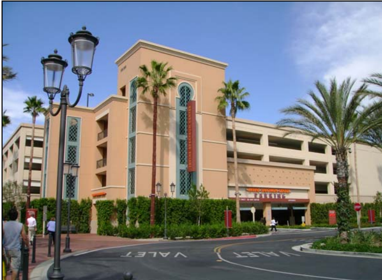
The Irvine Spectrum parking structure. Building mass is broken with various size openings, allowing for more light and safety. Color details and landscape enhance the functional look.
