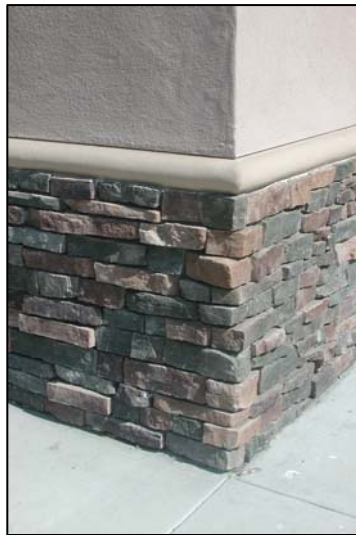
The unique surface texture and building details are carried around the corners of the building.
