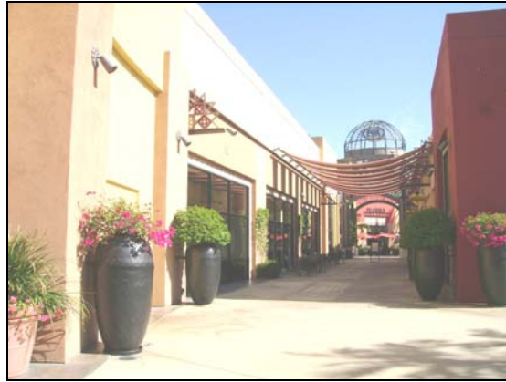
A paseo links different structures creating an outdoor plaza. It is further visually reinforced by the fabric overhang.
