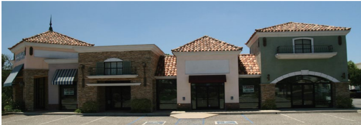
View of Building's East Elevation
