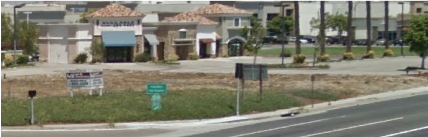
Northwest View of Existing Building
