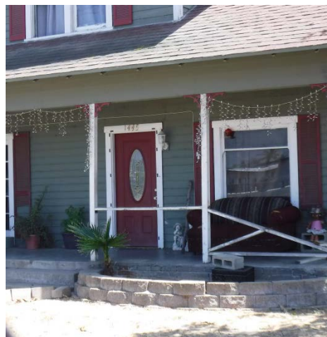
Primary Entrance, 1445 W. Mission Boulevard SOURCE: Sapphos Environmental, Inc., 2018
