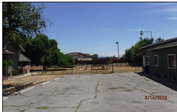
Site-View looking South towards Pool and Shade Structure
