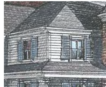
Multi-paned windows with shutters and lap siding.
