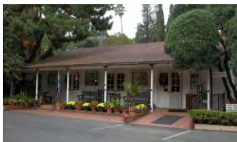
Simple one story massing with long continuous porch articulating entire front façade.
