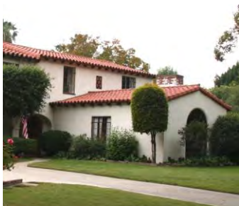
Contrasting dark brown fascia and window trim with pale stucco body and red "S" tile roof.
