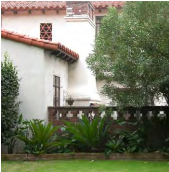
"S" tile roof with open eaves accentuated by decorative eave treatment and tile venting.
