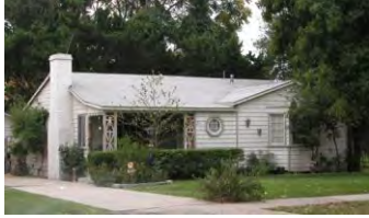
Long horizontal gable roof, with extensive use of lap siding and brick accent at chimney.
