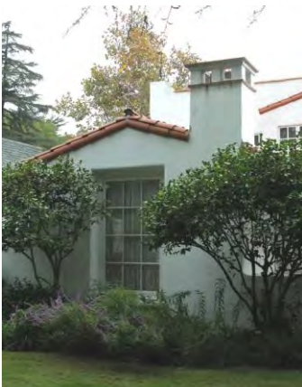
Tight rake with no exposed fascia, recessed feature window and decorative chimney cap.
