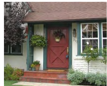
Covered Entry with decorative light fixture.
