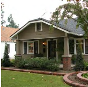
Covered porch with distinctive gable end treatment.
