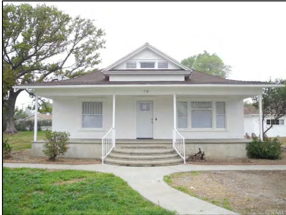
Residence-Front View looking north
