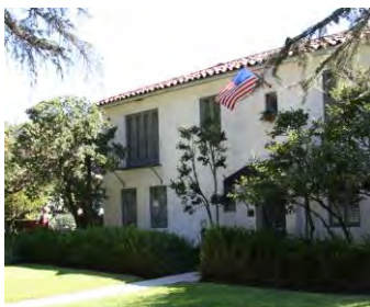
Simple Massing with Modest Wrought Iron Accents at Balcony and entry Awnings.
