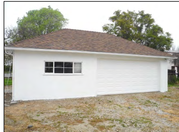
Detached garage with workshop View looking north
