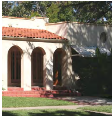
Arched recessed porch and shaped parapets.
