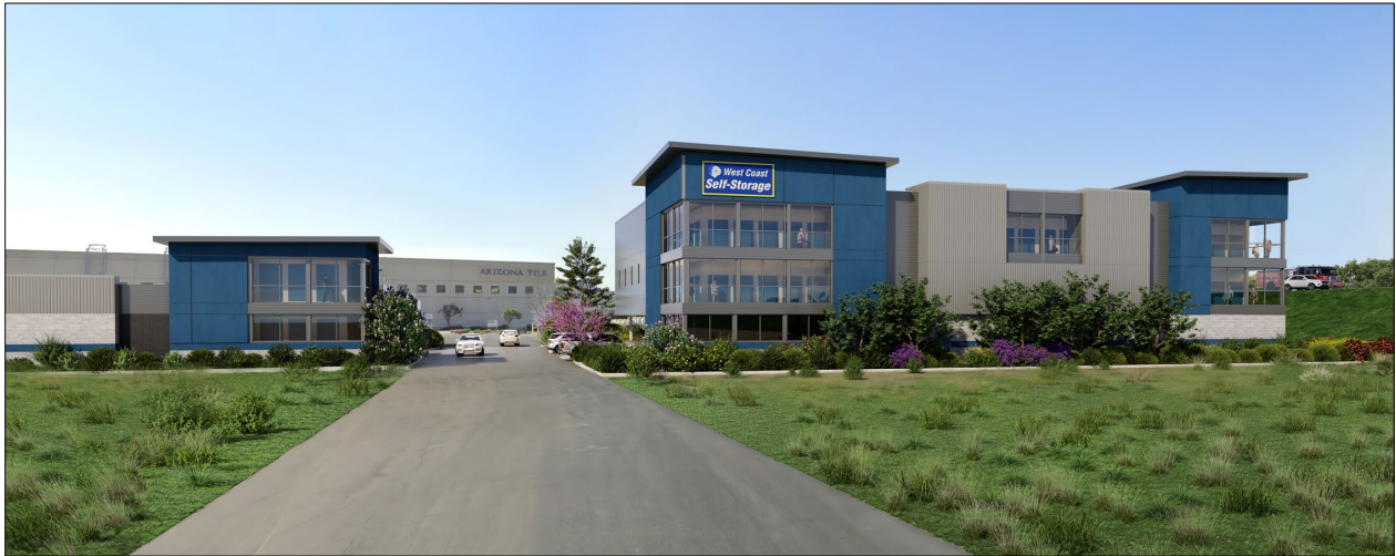
VIEW LOOKING SOUTH TO PROJECT AND ARIZONA TILE
