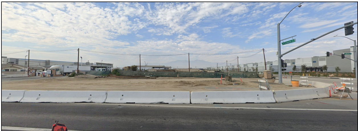
View from Merrill Avenue
