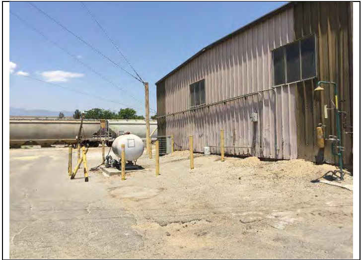
2. View of Warehouse Building (Building C)
