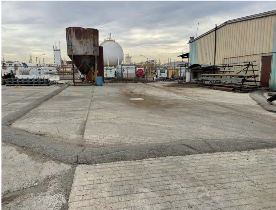
Photograph 3: Bermed truck-washing area by Building B.
