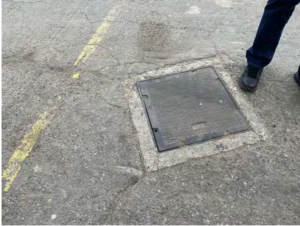
Photograph 11: Septic tank location by Building A.
