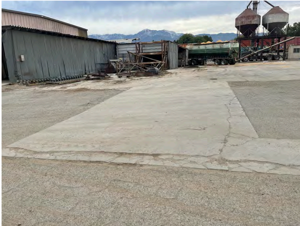
Photograph 7: Former underground storage tank area by Verhoeven Building C.
