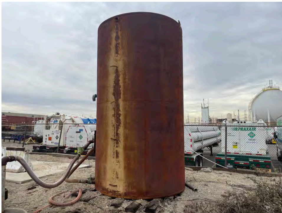
Photograph 2: Wash water storage tank by truck-washing area.
