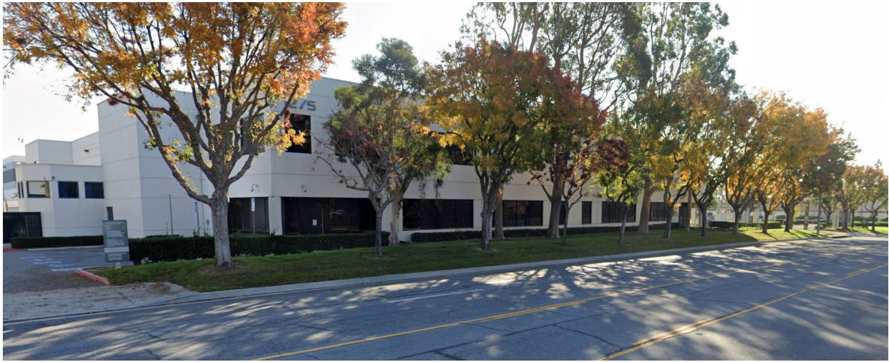
View looking southeast towards primary building.
