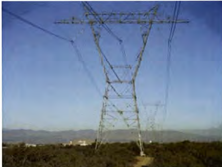
CA-SBR-8857H facing northeast.
