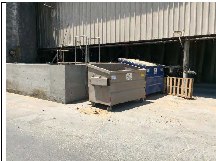
13. View of Trash Dumpsters
