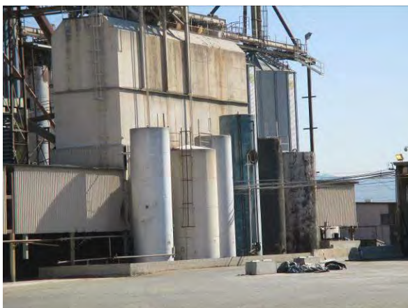
Photo #23 View of the ASTs containing molasses and fats.
