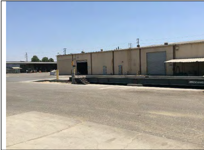
1. View of Main Building (Building A)
