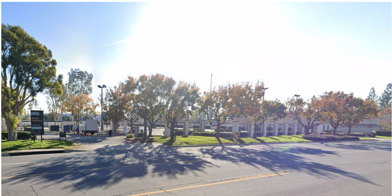
View looking southeast towards surface parking lot.
