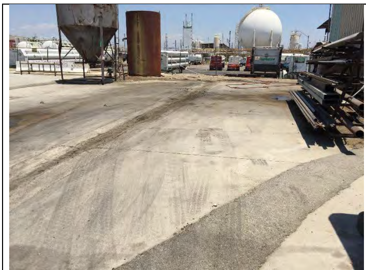
14. View of Former Vehicle Wash-Down Area
