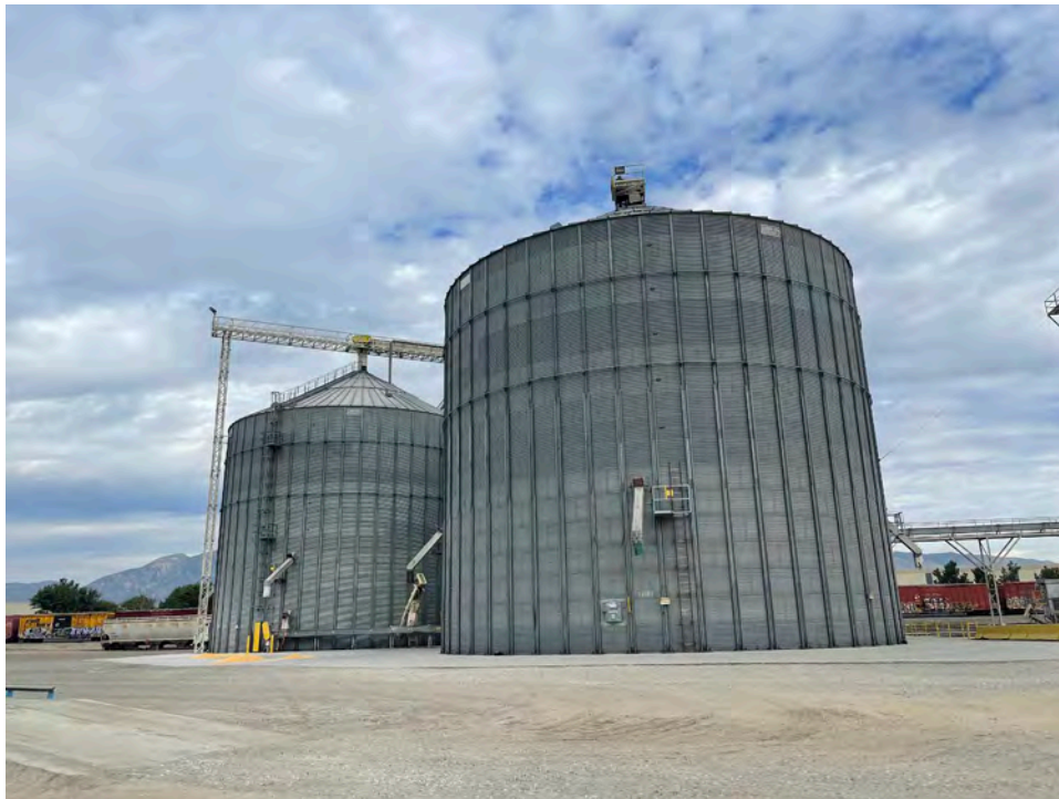
Photograph 10: Scoular grain storage silos.
