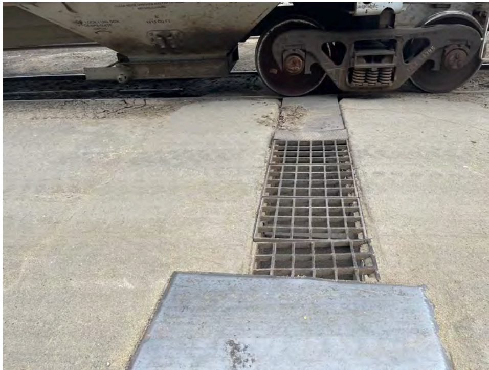
Photograph 12: Rail transloading area.
