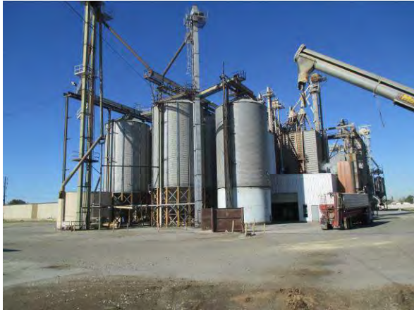
Photo #1 View of the mill located on the central portion of the site.
