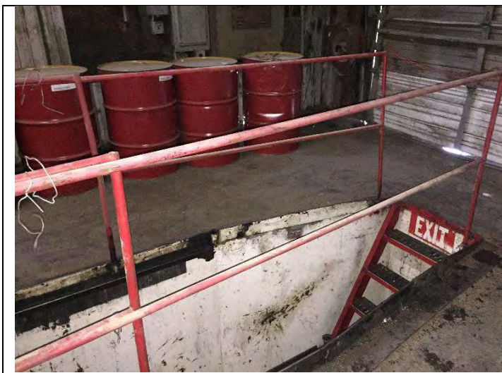
19. View of Service Pit within Building B
