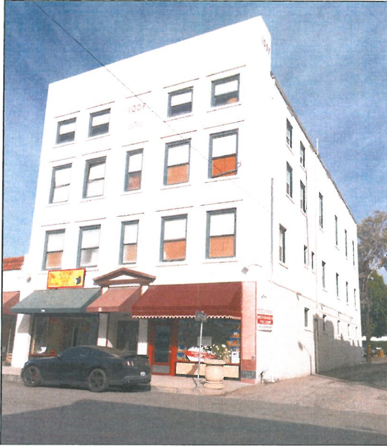
Front Façade and Alley (South Elevation)
