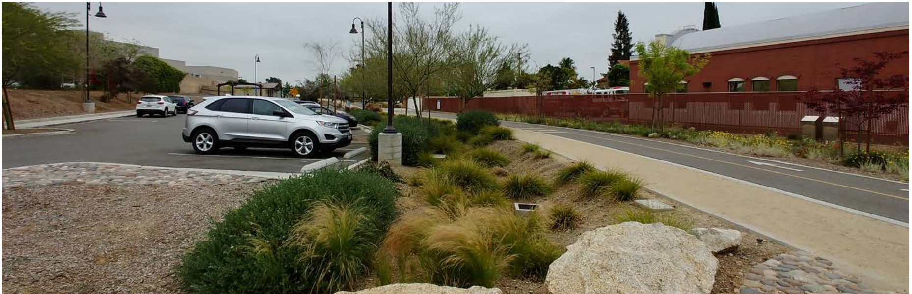
Rain garden, City of Brea
