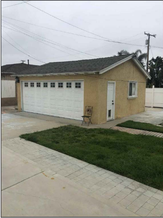
View facing southeast
