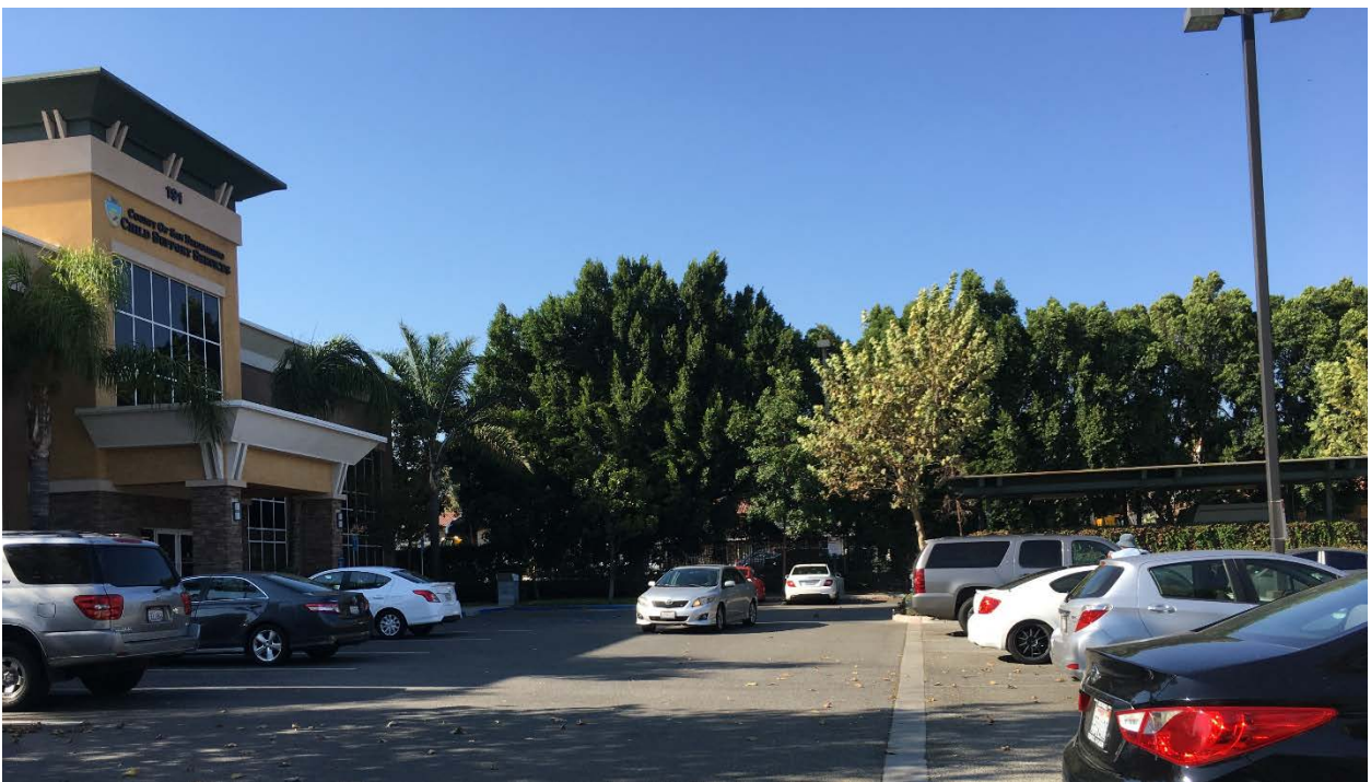
View of County Building from project site, looking northeast
