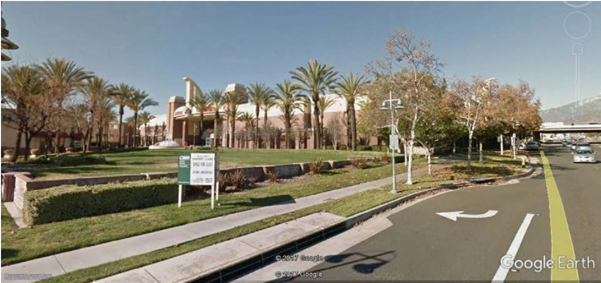
VIEW OF THEATRE AND PARK SPACE (FUTURE RESTAURANT PAD), LOOKING NORTHWEST
