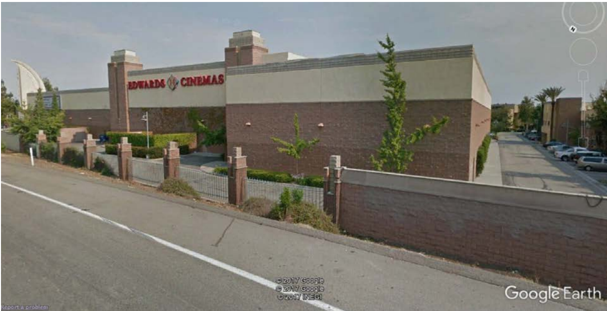
VIEW OF REAR OF THEATRE, LOOKING SOUTHEAST
