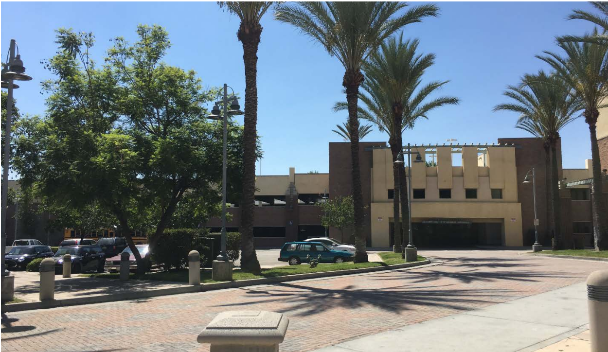
VIEW OF PARKING STRUCTURE, LOOKING WEST
