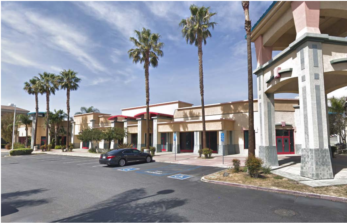
View of the suite, facing northwest
