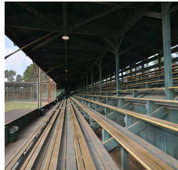
Figure 8. Jay Littleton Ball Park, east wing of the grandstand.
