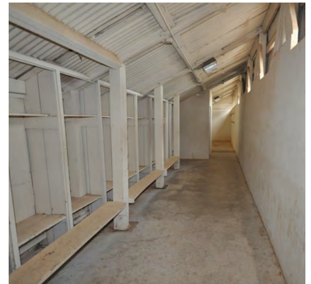
Figure 9. Jay Littleton Ball Park, locker room.
