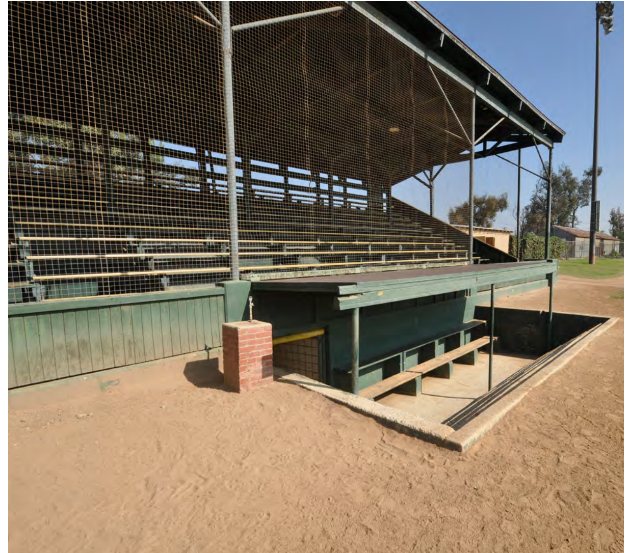
Figure 10. Jay Littleton Ball Park, looking towards the dugout near third base.
