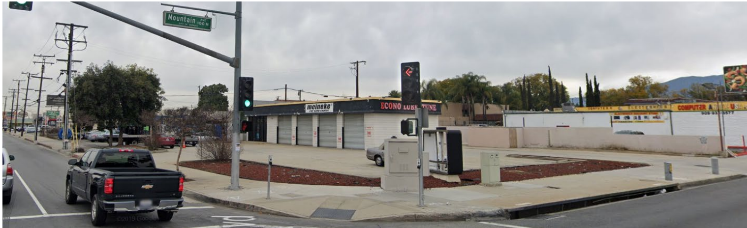
NORTHWEST CORNER VIEW OF HOLT BLVD AND MOUNTAIN AVE
