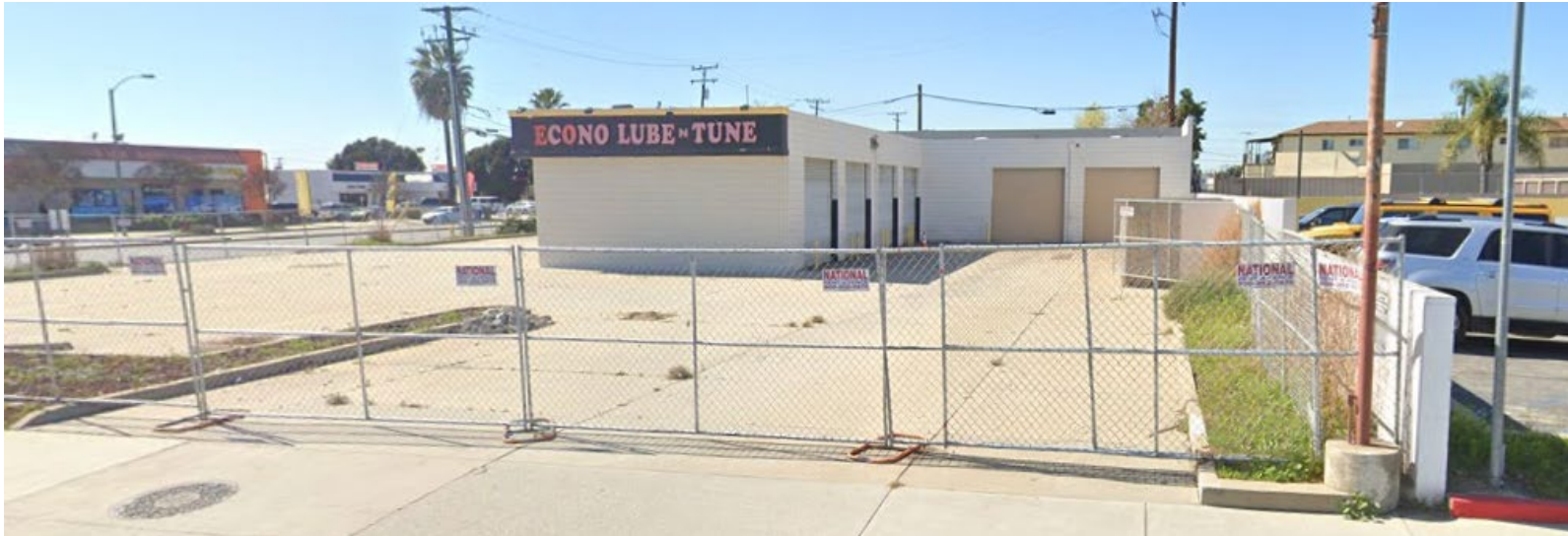
NORTHEAST VIEW OF EXISTING BUILDING TO BE DEMOLISHED
