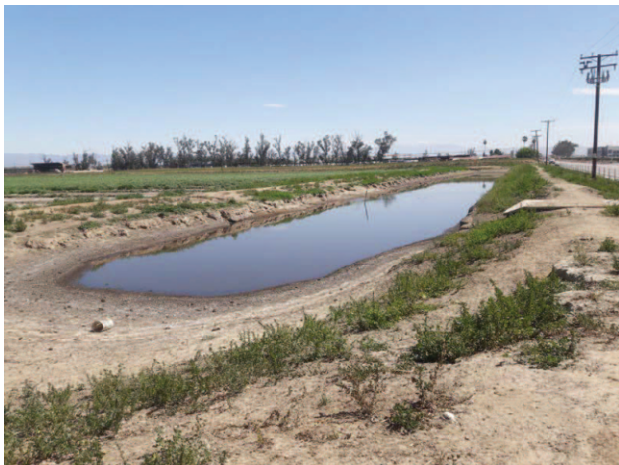
View of wastewater lagoon.
