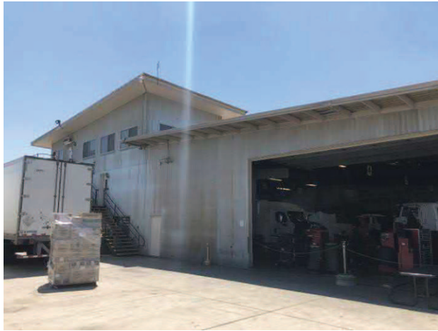
View of truck service building and office.
