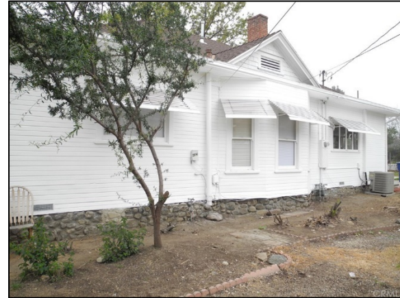
Residence-Side View looking northwest
