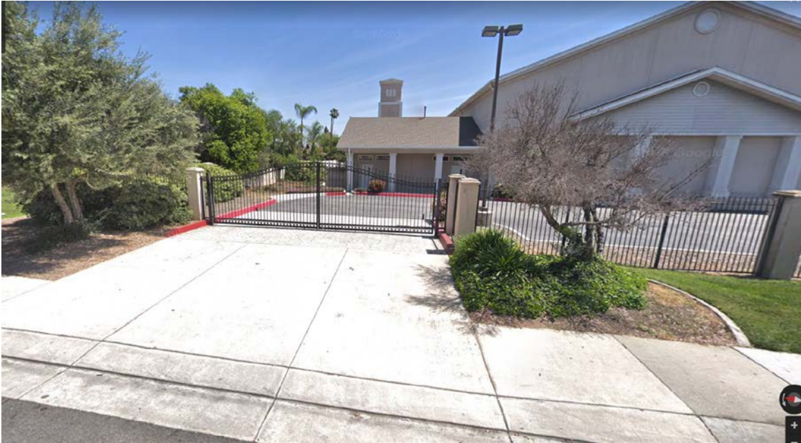
Church's Northwest Driveway – Looking East from Virginia Avenue
