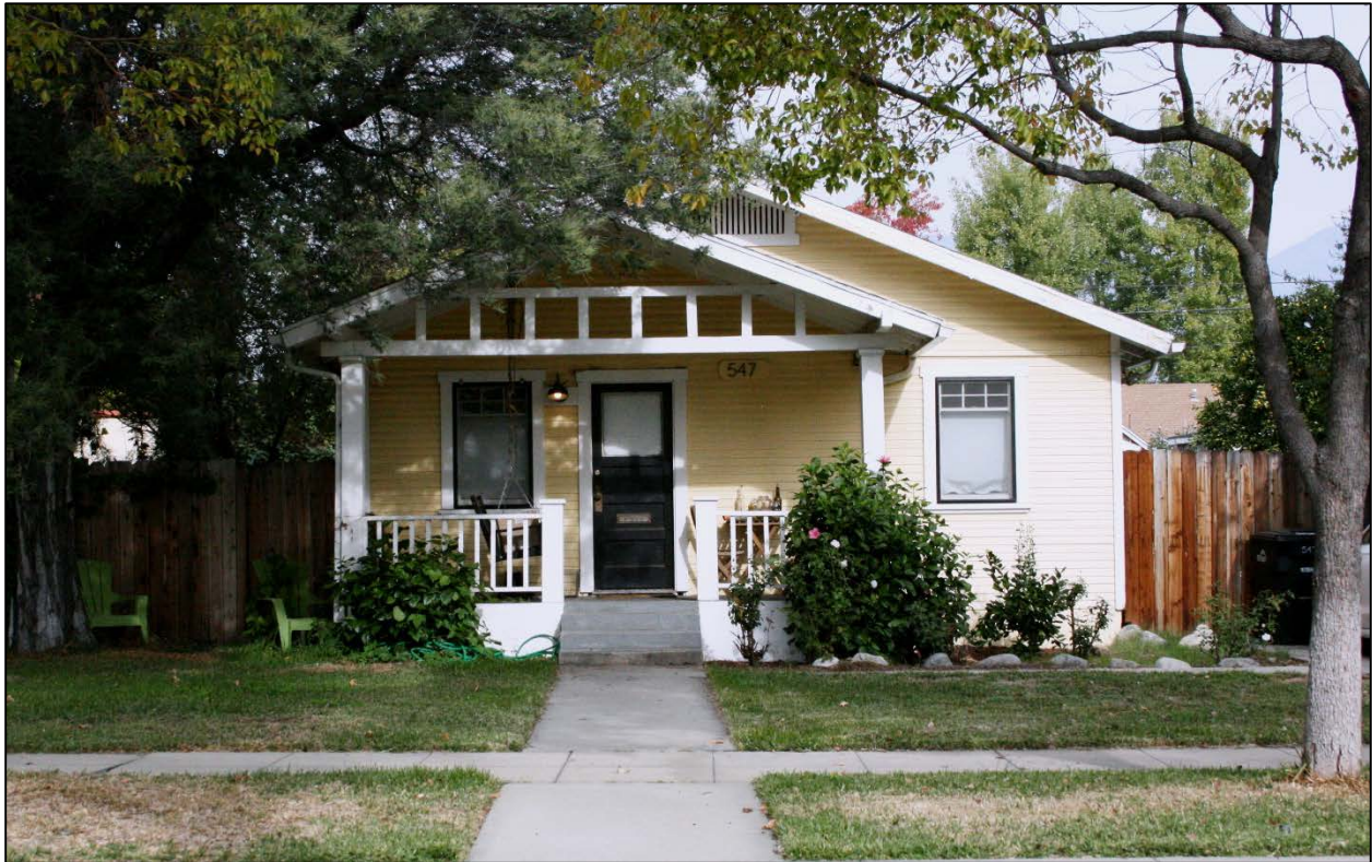
View looking north
