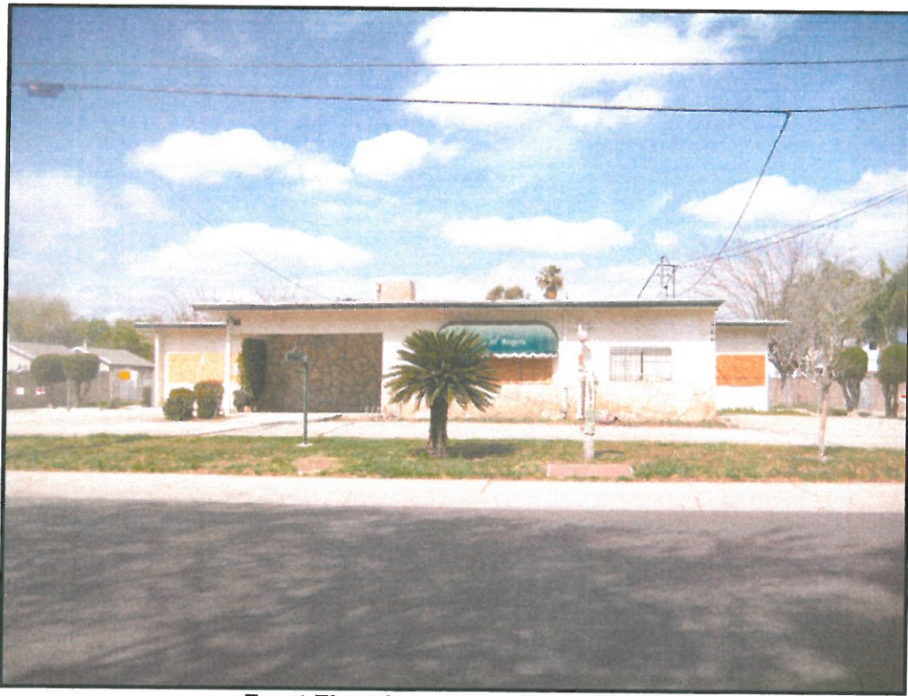
Front Elevation – From Maple Street
