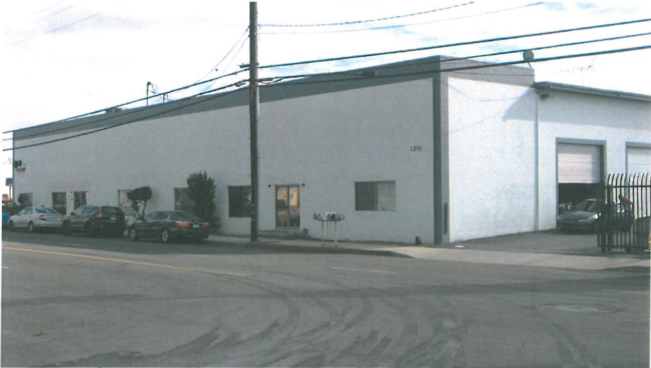
Building's North Elevation
