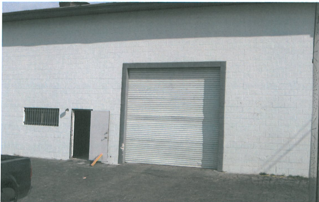
Office Entrance & Roll Up Door (West Elevation)
