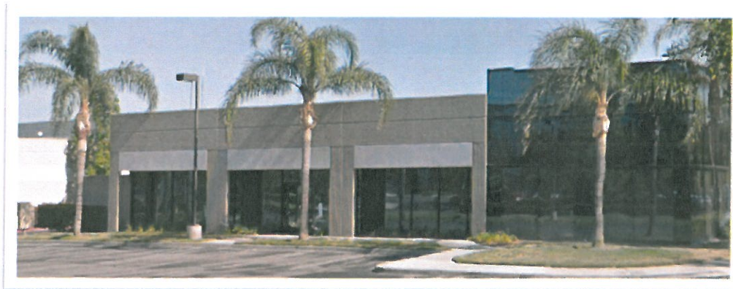
Project location, exterior and adjacent units (North).
