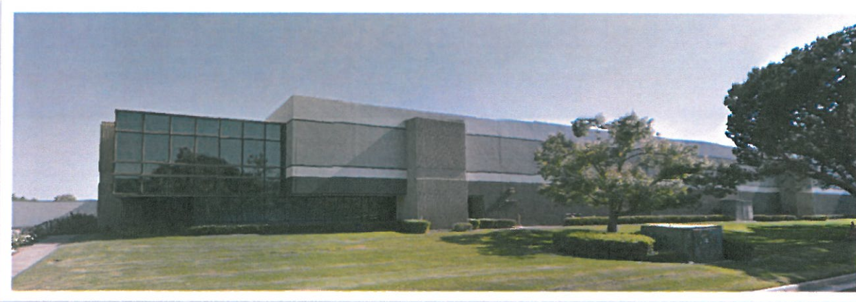
Site to the east of the project location.
