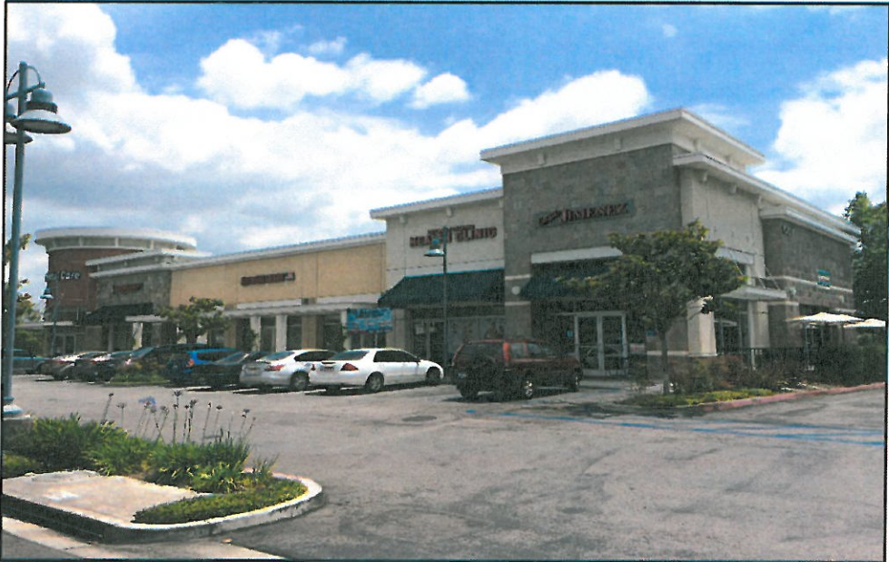
Project location, adjacent tenants.
