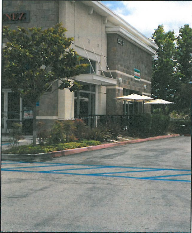
Project location, outside patio area.
