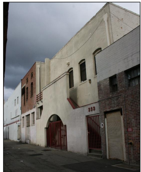
Rear of Building (West Elevation)
