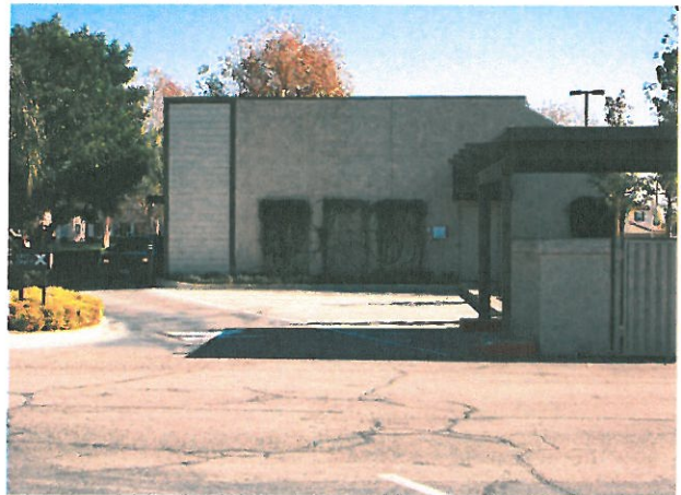
West Elevation of Project Site
