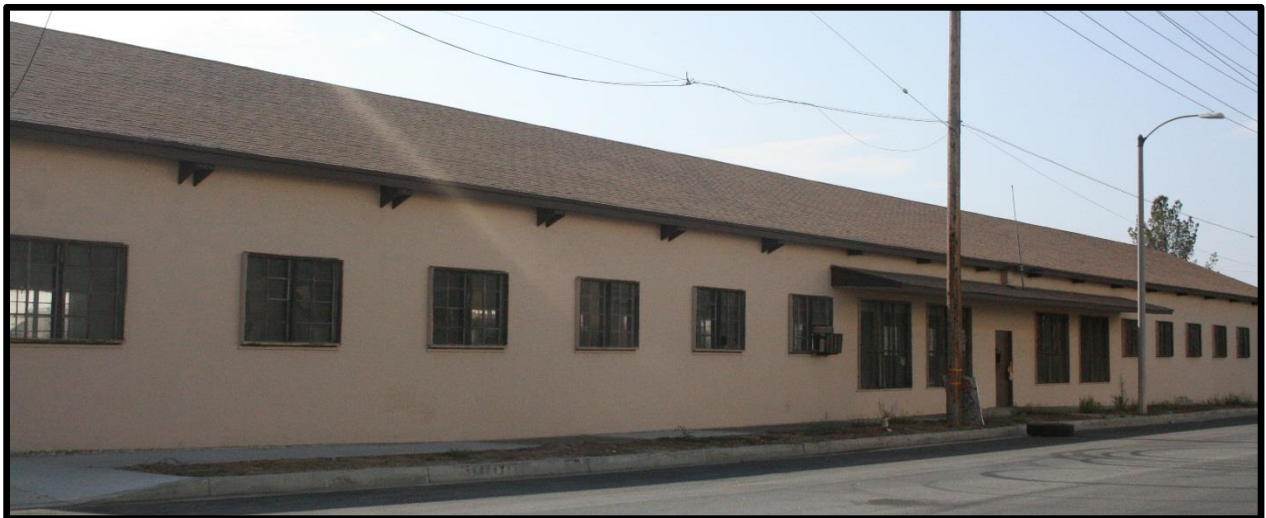
View looking east at project site.
