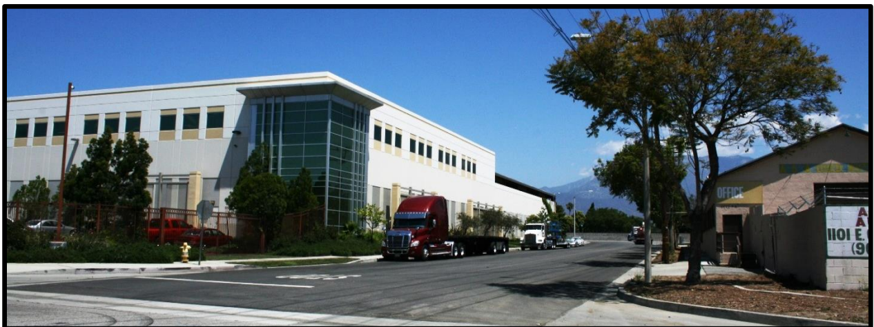
View looking west at existing industrial building
