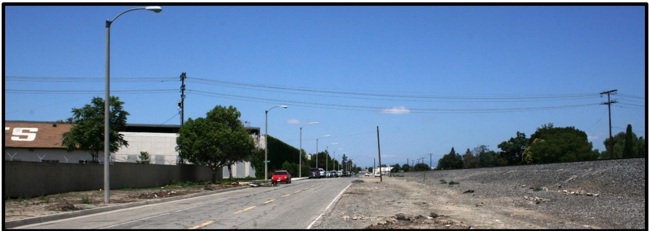
View looking north at existing railroad corridor
