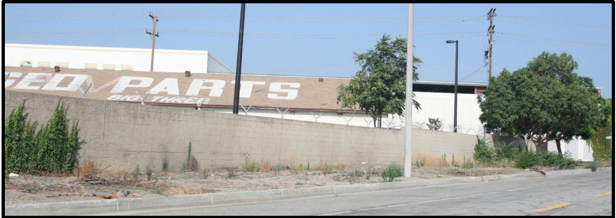
View looking southwest at project site.
