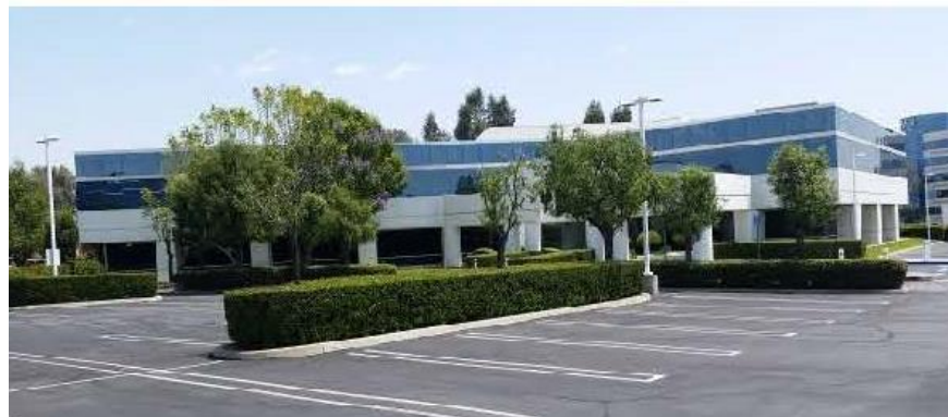
2-Story Office building within the southern portion of the Project Site
