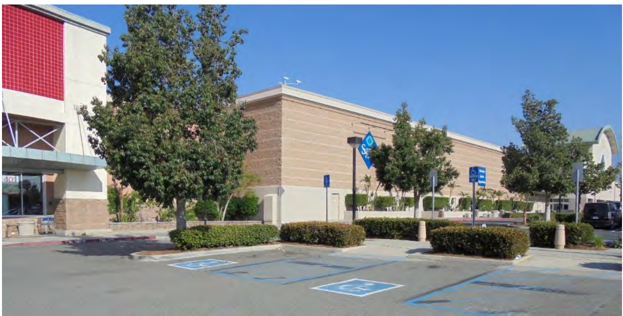
Existing Commercial Store North of Project Site (Sam's Club)
