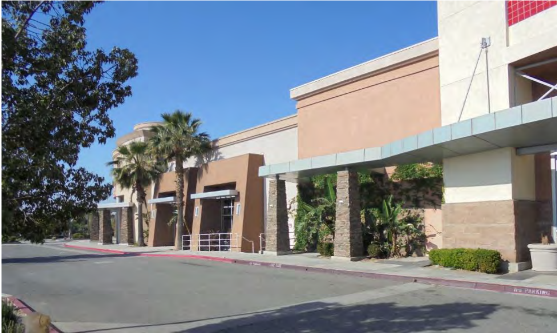
Existing Commercial Store South of Project Site
