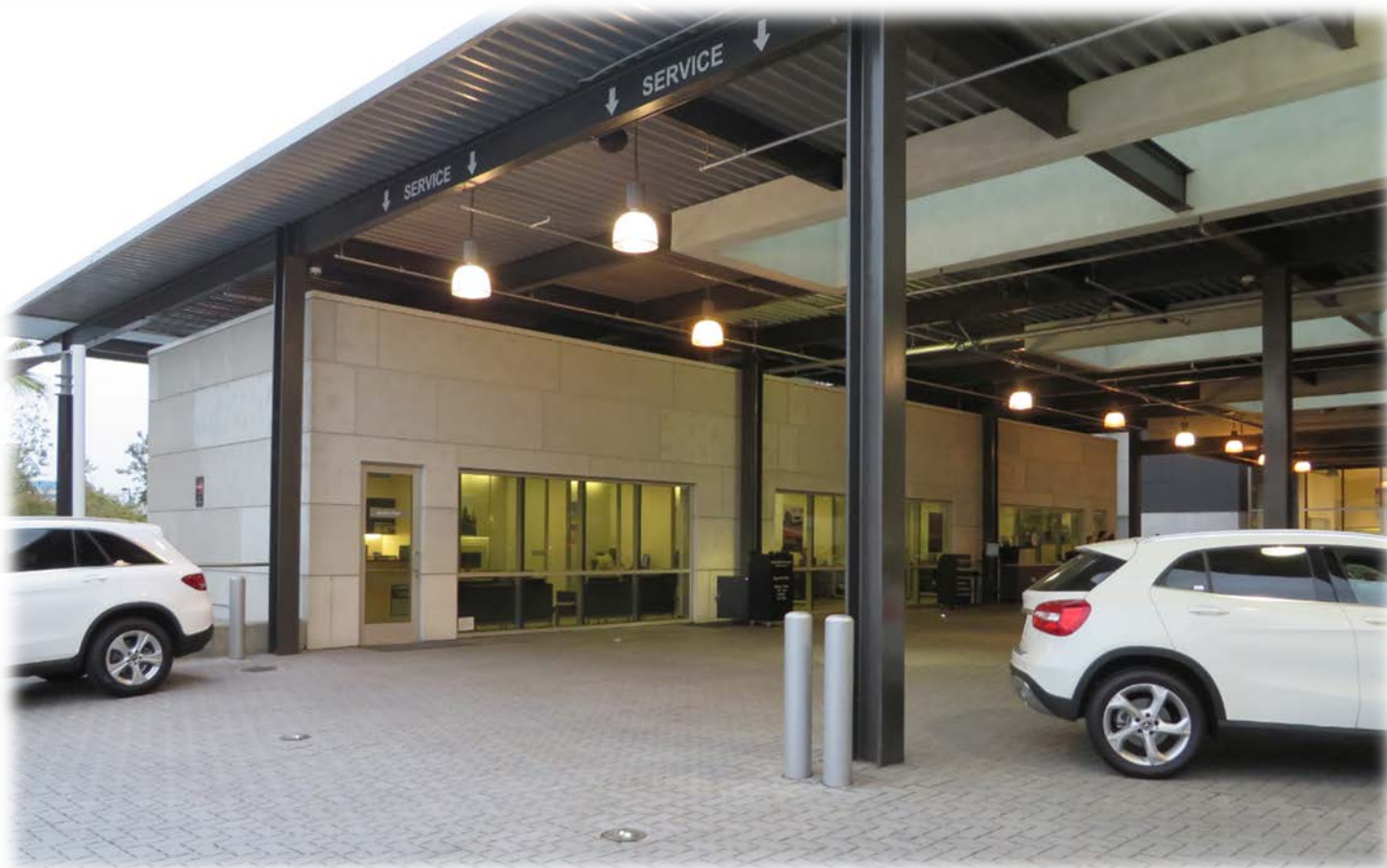
East Elevation of Existing Service Area Offices
