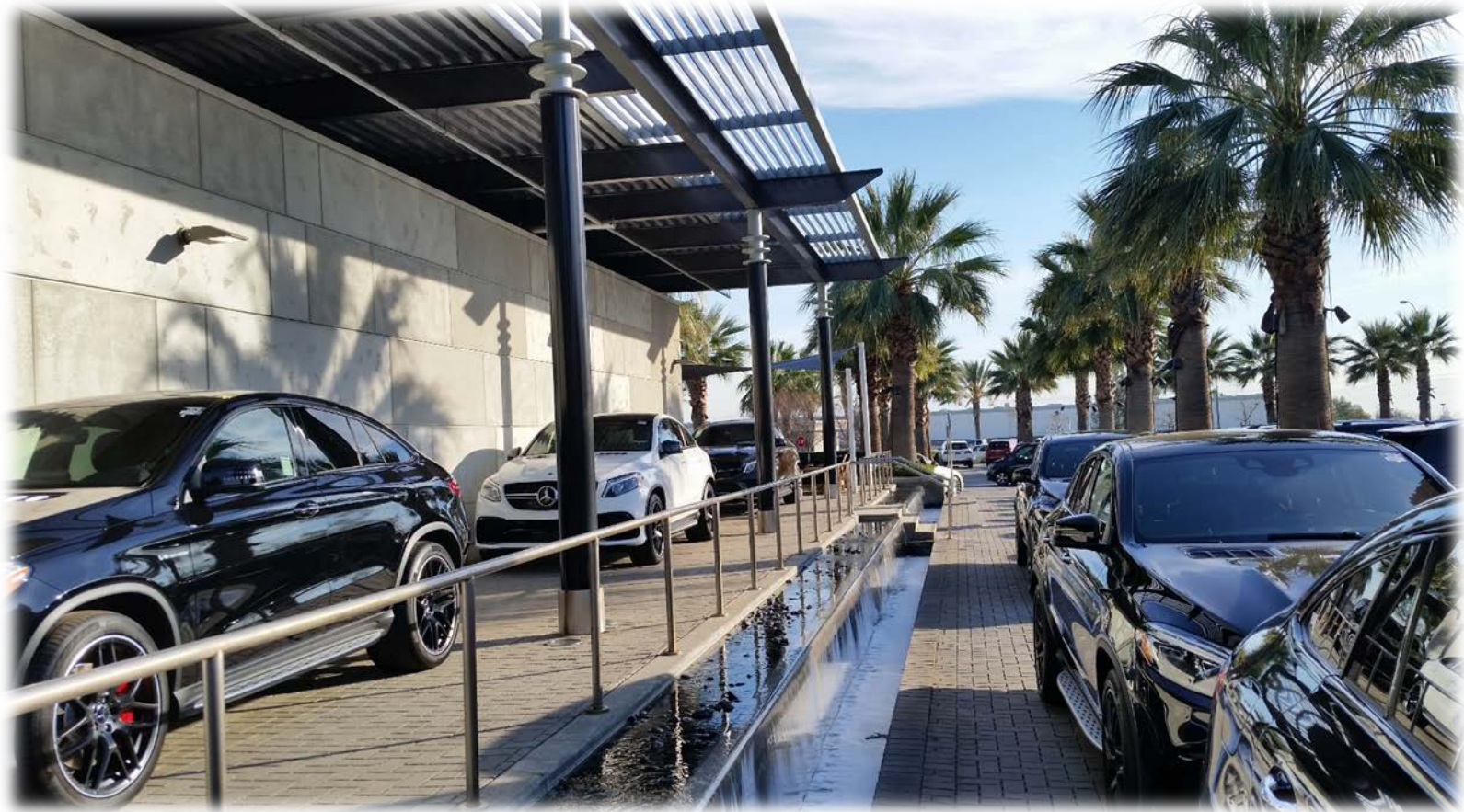
Side View (West Elevation) of Existing Service Office Area
