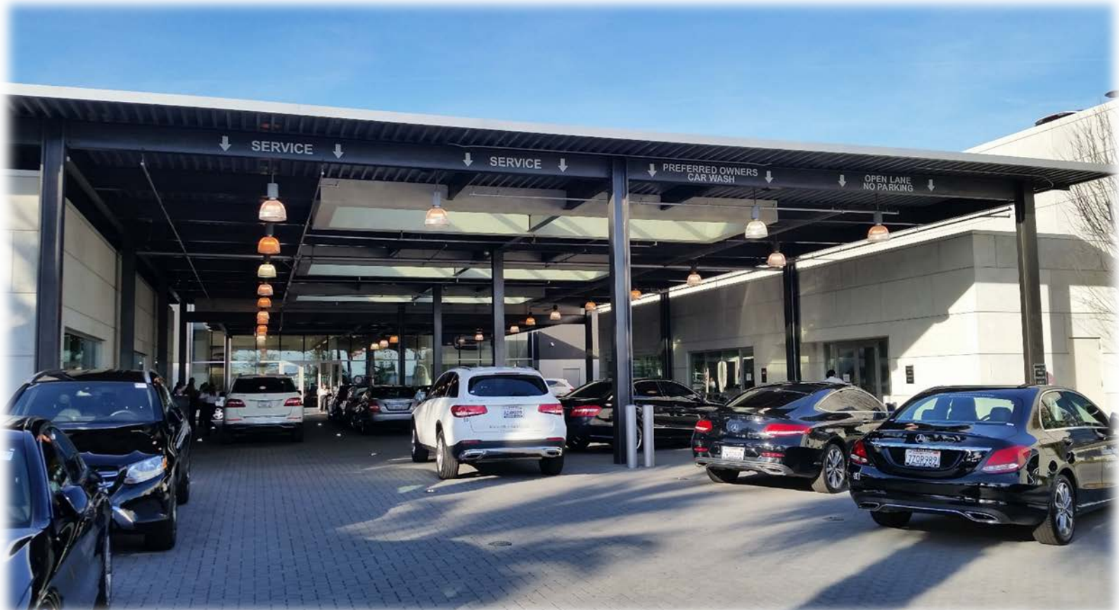
View of South Elevation of Existing Service Area
