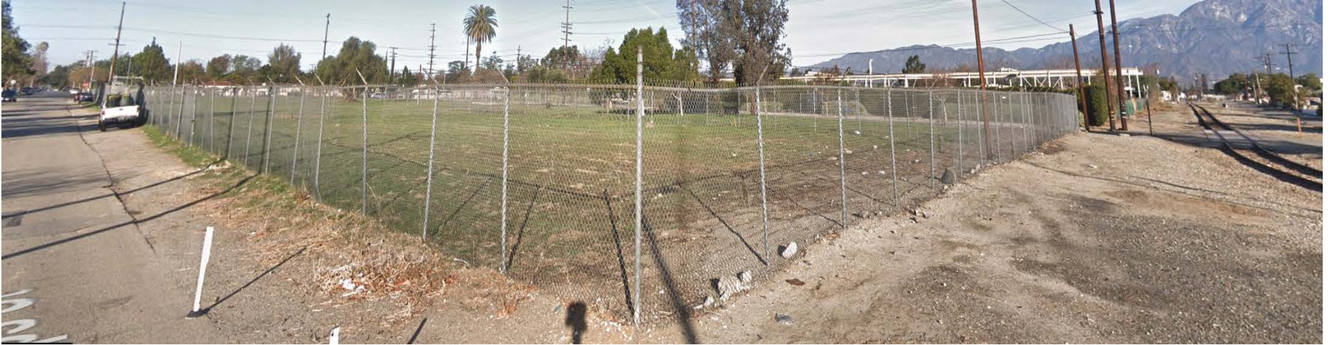
SOUTHEAST CORNER VIEW OF PROJECT SITE (Phillips St & Railroad Tracks)
