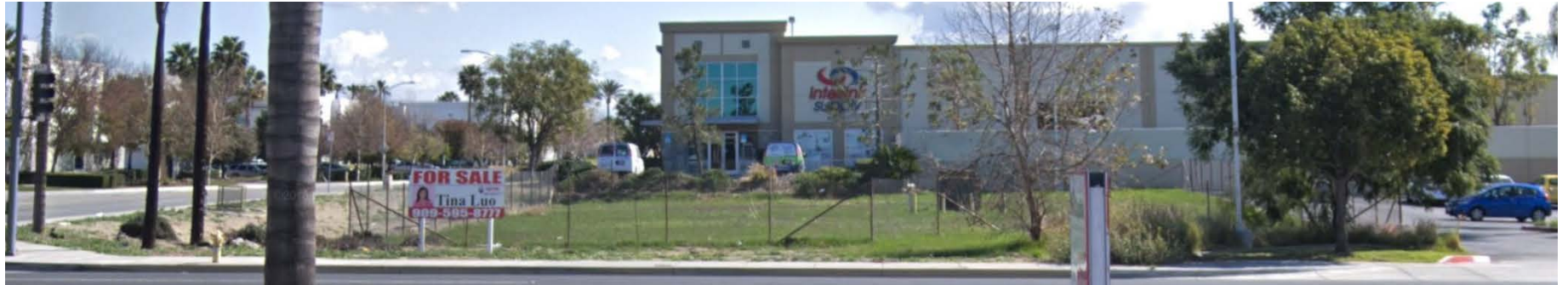
VIEW LOOKING EAST FROM GROVE AVENUE
