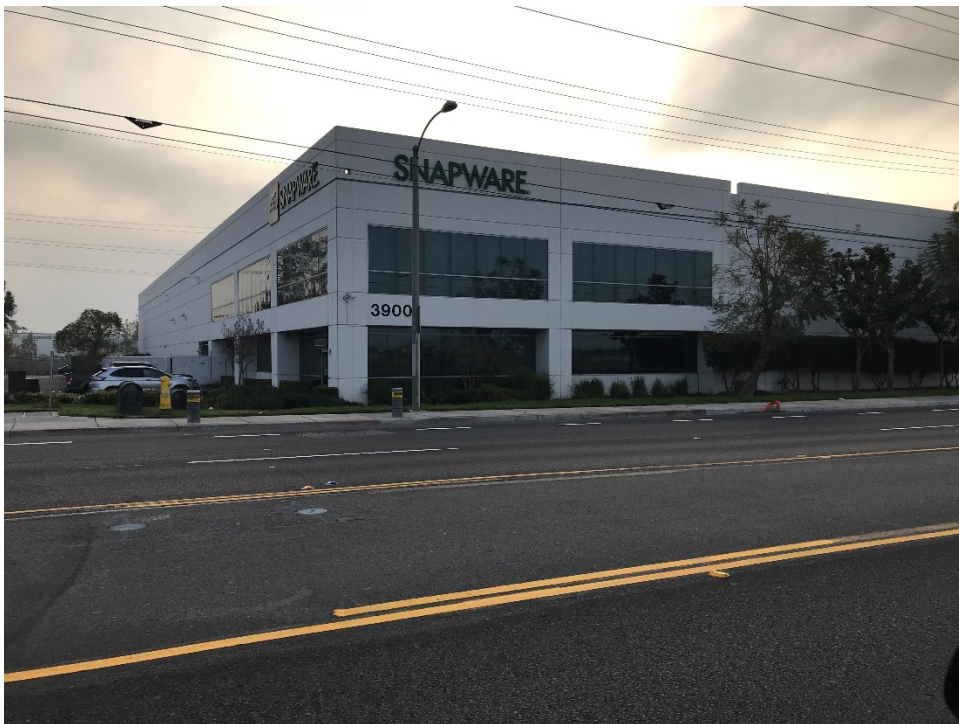
Photo 12 – Snapware building to the east of the Property.
