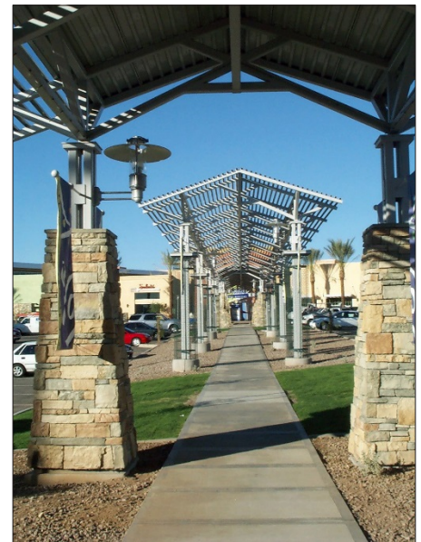
Connecting Walkway with Trellis
