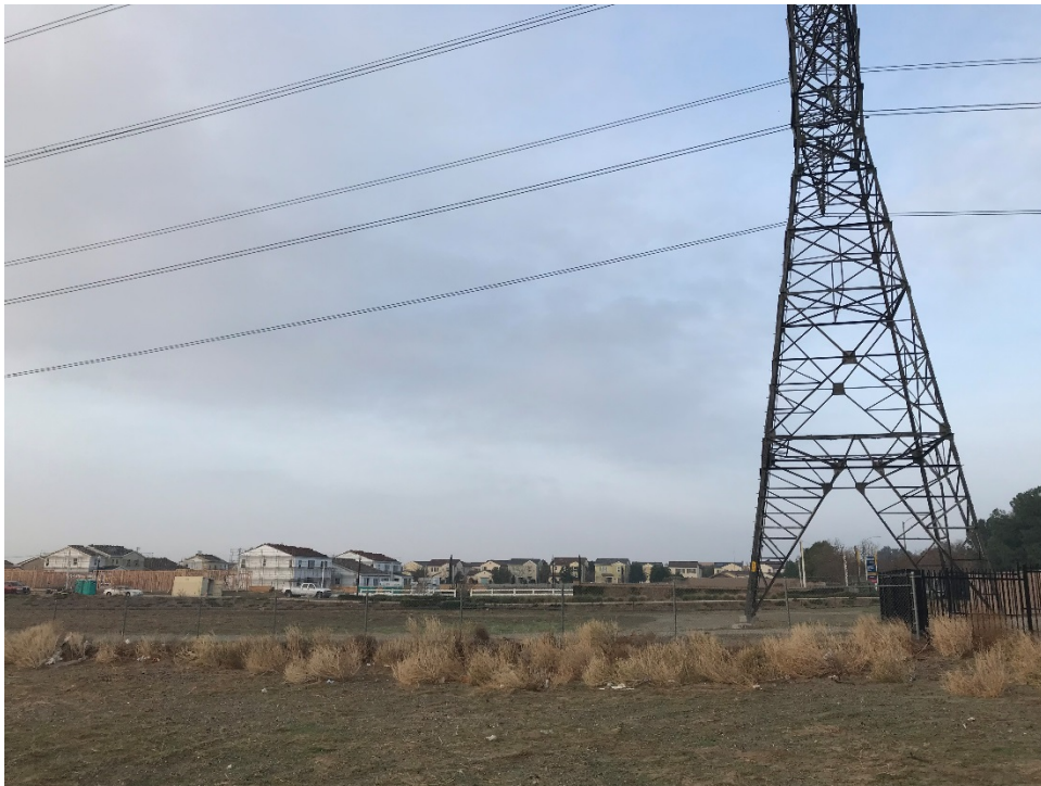
Photo 10 – High-tension electrical lines adjoining the Property to the west.
