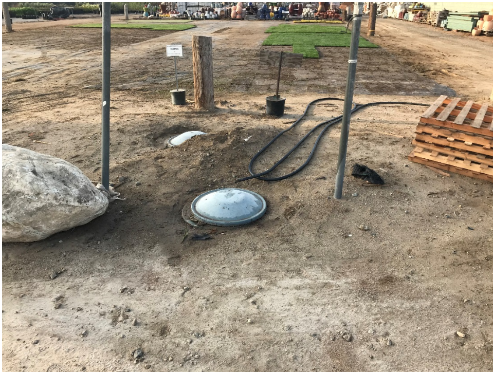
Photo 28 – Septic system on the south-central portion of the Property.
